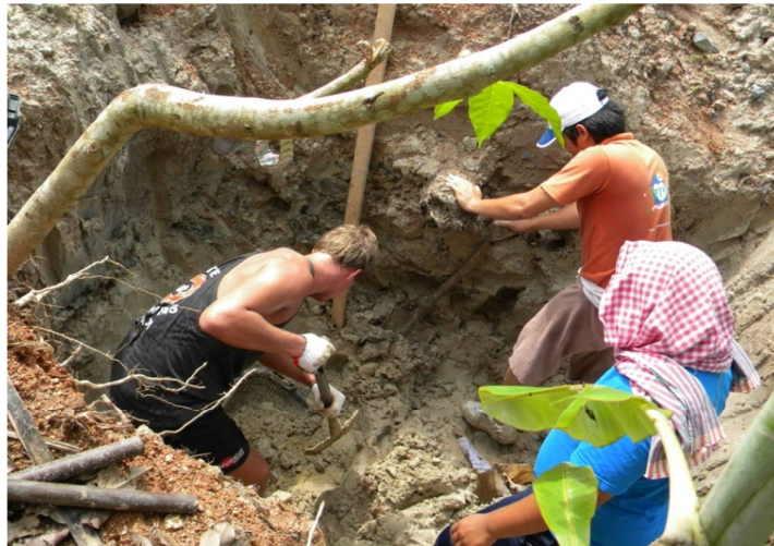
(f) Constructing the new building for the bakery and coffee shop
