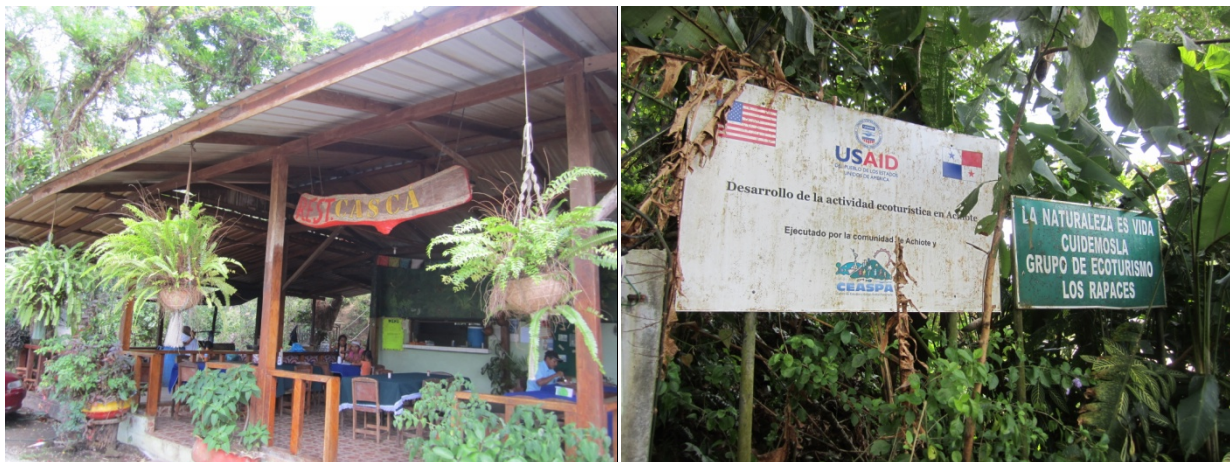
Figure 4.3. Photographs of the restaurant built in Achiote as part of the community ecotourism initiative with CEASPA and USAID
