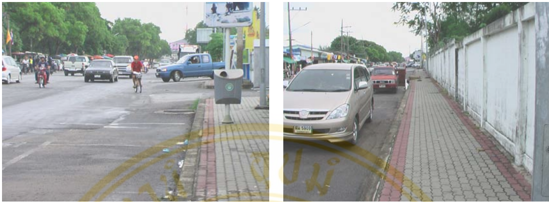
Figure 4.4 Road conditions and sidewalks at Kaoseng Road.
