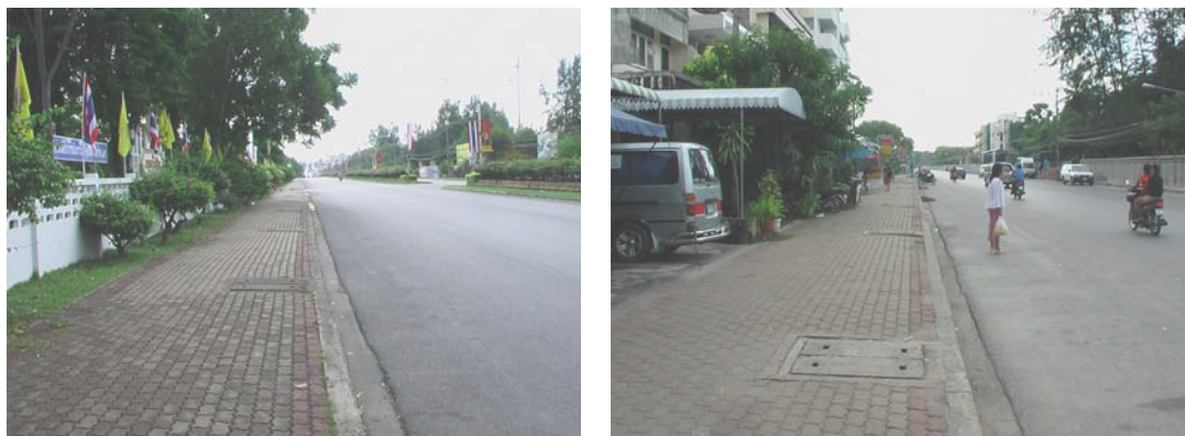
Figure 4.6 Sidewalk conditions and Rachadamnoen Road.
