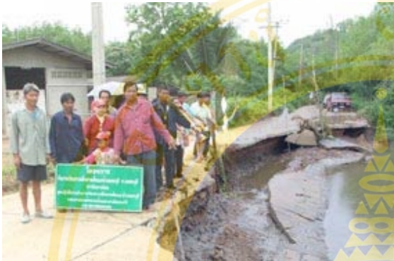
Figure 5.1 Broken concrete road at the entry way (Picture from Matichon, 8/9/2005)
