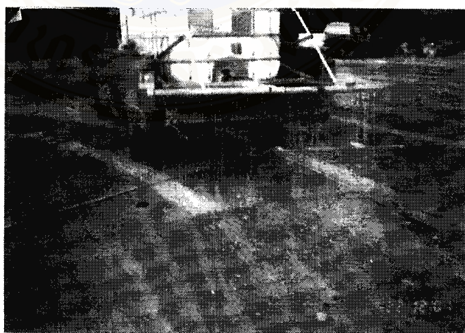
Figure 5-3 Water spraying around the parking area
