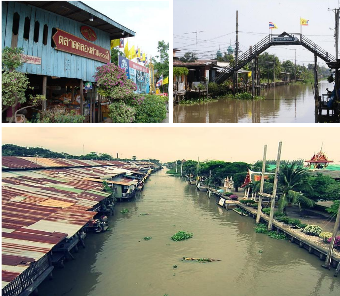
Figure 2.7 Riverside View of Klong Suan Market
