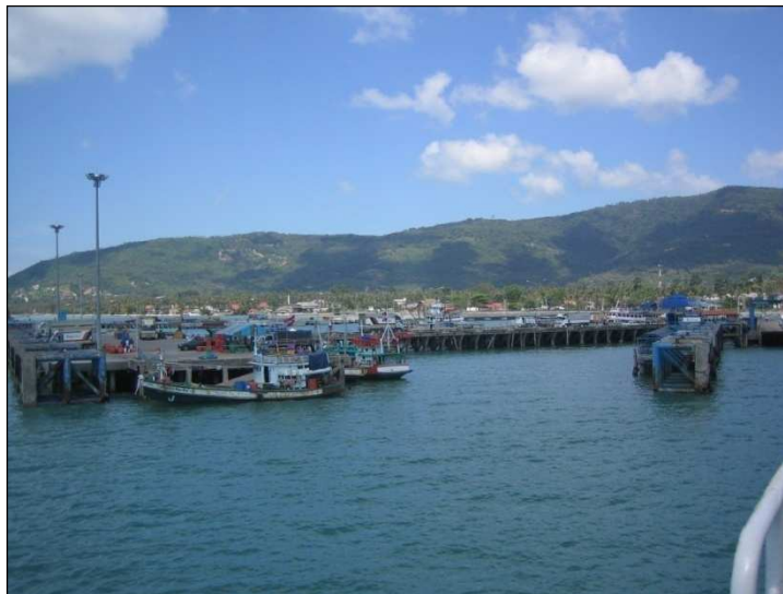
Plate 6.4: The Nathon pier, where the ferry connects to the mainland
