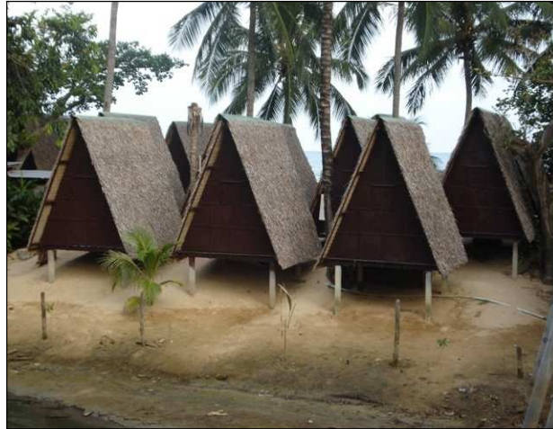
Plate 6.11: Some of the very first bungalows on Lamai Beach
