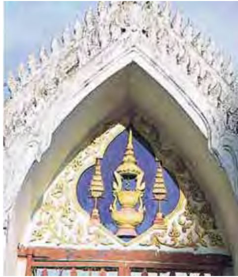
Figure 19: Royal seal of King Rama IV at the entrance of Phra Prang Source: Photograph book of Wat Arun Ratchawararam : 1991
