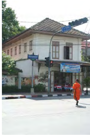
Figure 106: The existent old building
