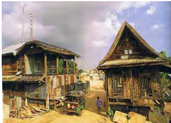
Figure 104: Vernacular houses which were demolished due to Arun Aummarin Road expansion
