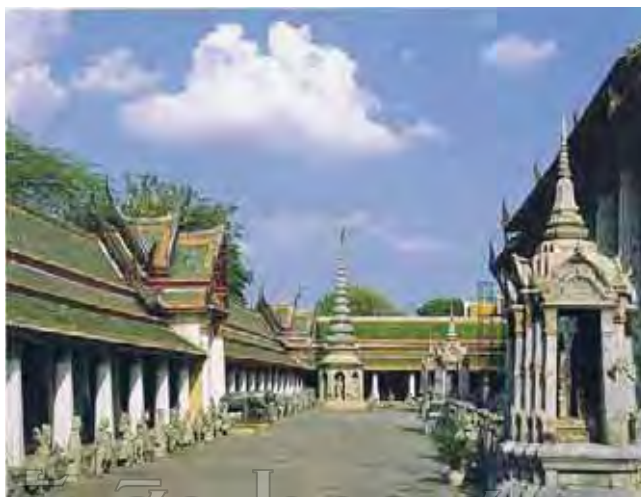
Figure 49: The peripheral balcony and surrounding architectures Source: Photograph book of Wat Arun Ratchawararam : 1991
