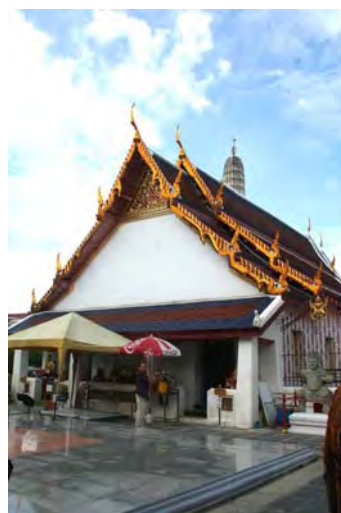
Figure 97: The pavement in front of Viharn-noi or the small chapel after adaptation
