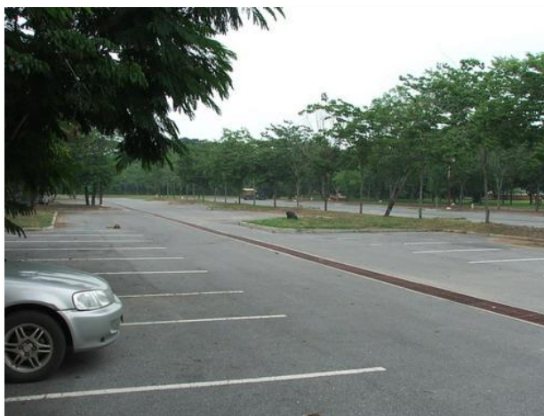
Figure 20 Parking area behind the Tourist Information Centre. Only a few cars or coaches use this parking area
