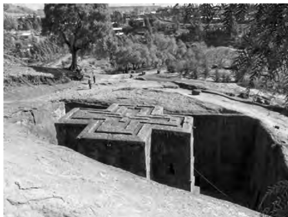
Photo 2: The Giorgis Church at Lalibela: excavated in Greek crucifix form and 12 m in length, width and height.
