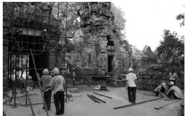
Photo 2. WMF team constructing scaffolding for emergency consolidation of western gate, Preah Khan.
