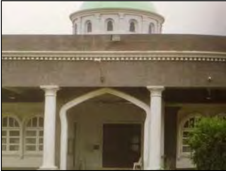
Figure 66: Ansorissunnah royal mosque
