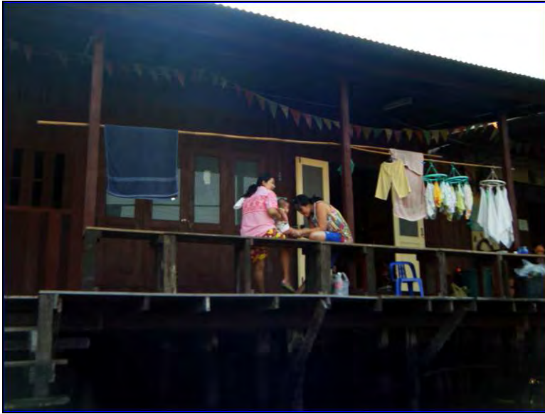
Figure 3: Sample picture of Villager House on Bangkok Noi canal
