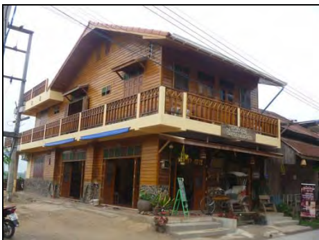
Figure 52 Newly built two story wooden house, exposed two sides Source: Photograph taken by author on 26 February 2011
