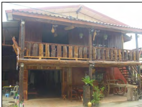
Figure 59 A newly built wooden house with big flat rails around veranda Source: Photograph taken by author on February 26, 2011
