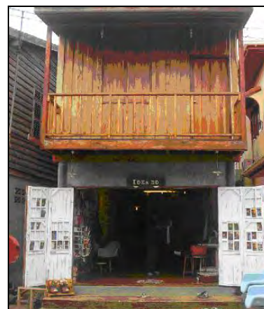
Figure 47 Two-story wooden shophouse, repaired recently
