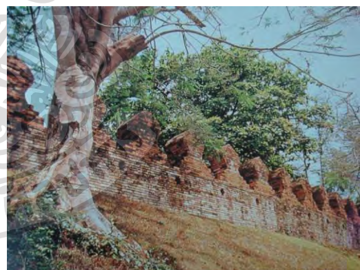
Figure 26 The north-eastern section of the walls of Nakhon, with bai sema crenellations.
