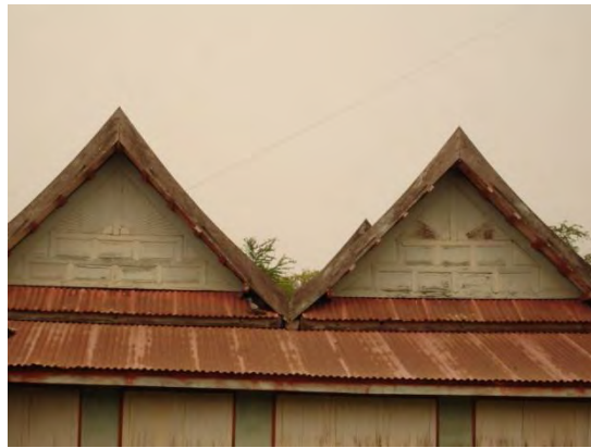
Figure 252: Thai style gable roof
