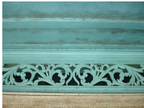
Figure 150: Ventilation panel in shophouse
