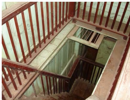
Figure 156: In gallery, between 1 st floor and 2 nd floor has sliding security round steel bars and wooden frame door which can lock with a stair to prevent risk from thief.
