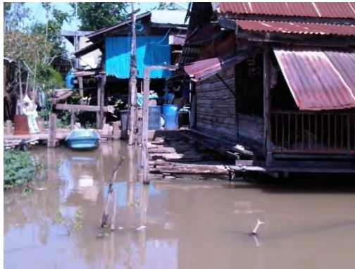
Figure 225: Bamboo floating structure raft under the house
