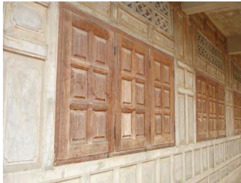
Figure 114: Thai style timber wall
