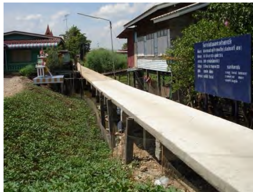
Figure 262: Concrete path in Zone C, width of the path is approximately 1.5 meters (All photos in Figure 255-262 were taken by Buatham, O., 2012)
