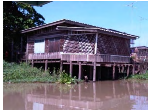
Figure 181: Timber house with trellis shading
