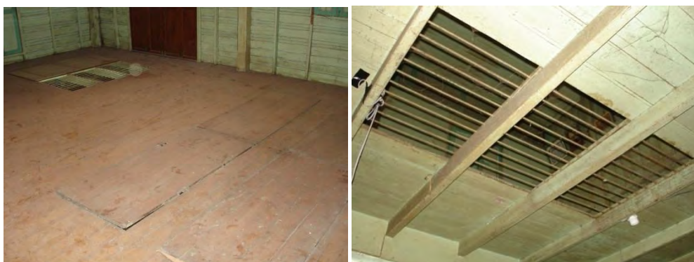
Figure 157: Some part of timber floor on 2 nd floor has security round steel bars; can open to look down to the 1 st floor.
