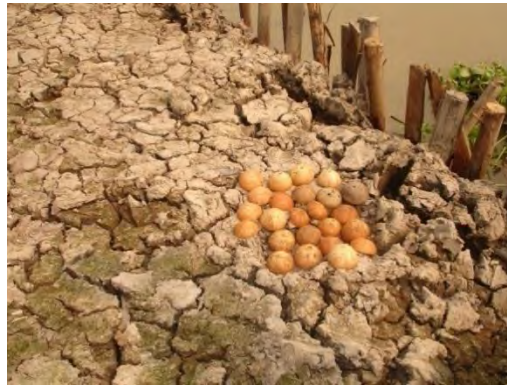
Figure 314: Use of coconut shell to protect soil erosion on flood damaged landscape. (photo taken by Buatham, O., 2012)
