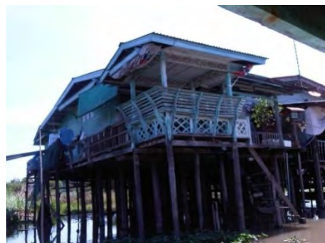
Figure 178: Typical Thai style house and terrace raised on stilts.
