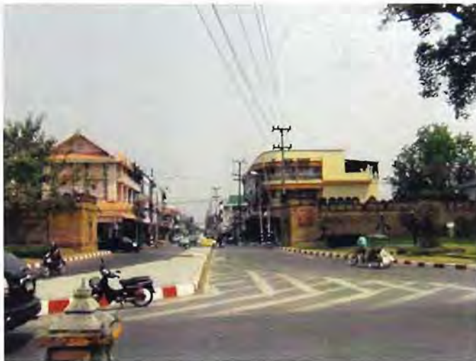
Figure 79 : Suan Prung Gate, Chiangmai City Wall, by the author on 19th March 2011
