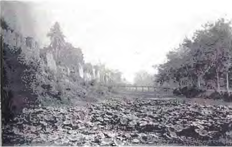
Figure 2 : Chiangmai City Wall in the past
