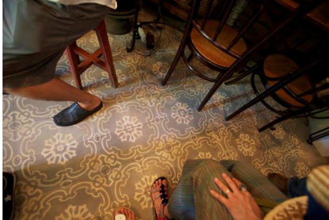
Figure 59: Original tiles had been revived back to the original by a professional manner of cleaning and retreating, Source: Naratuschan N.
