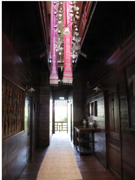
Figure 204: Compared with the Figure 203 above, we can notice that the corridor width is much narrower than earlier (to expand the size of the rooms), Source: Suparee B.
