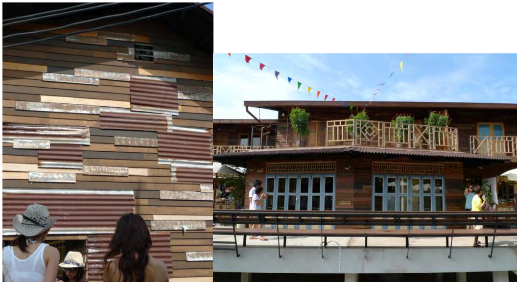
Figure 139: The concept of “old form + new materials” was chosen to develop the replicating Hua Hin old market community at Plearnwan, Source: Naratuschan N.
