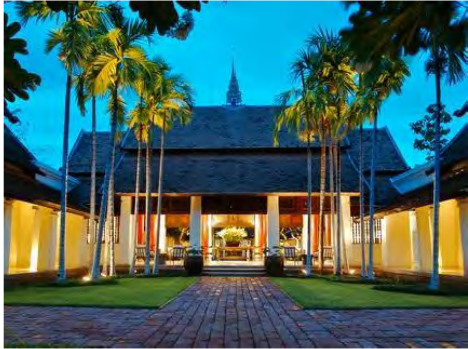
Figure 116: Rachamankha hotel, inspired by the local northern temple architecture and blended with various aspects of the culture, creating a world class architecture, Source: Rachamangka website
