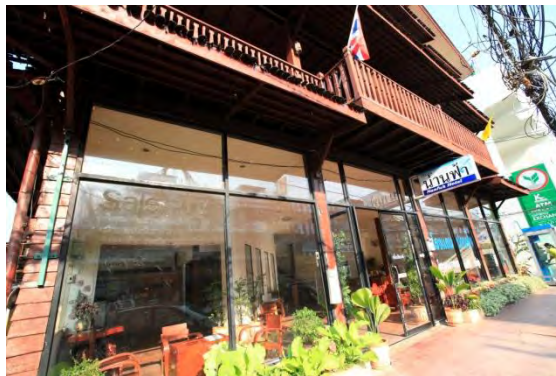
Figure 181: 1 st floor, the photo was taken on the last day before the renovation got started, Source: Narin
