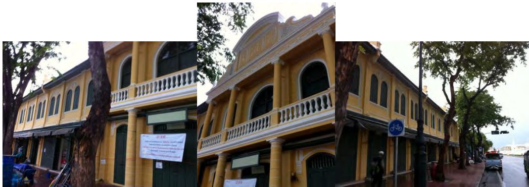
Figures 285-287: The colonial-style buildings on Na Phra Lan, Source: Naratuschan N.
