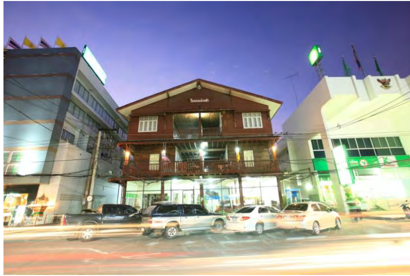
Figure 171: Nanfa hotel kept this look after the second renovation for more than 50 years (this photo had been taken at January 2010 two days before renovation). It is located beside Kasikorn Bank (Nan Province branch) on Sumon Dheveraj Road. Source: Narin N.
