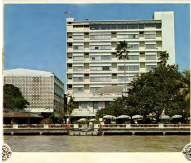
Figure 32: The Oriental Hotel in 1970s. Two buildings had been built to serve more customers, the tallest behind is “River Wing”, the one on the left is “Tower Wing”, and in the middle is the ‘ Authors Residences ’ (“Authors Wing”). Source: ThaiDVD.net (2010)
