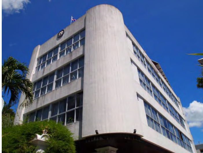
Figure 102: The Puck-Sa-Va-yu-puck sign stands on top of the building to represent the property ownership of Treasury Department under Ministry of Finances, Source: Naratuschan N.
