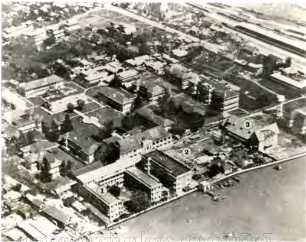
Figure 39: Development of Siriraj Hospital, 1952
