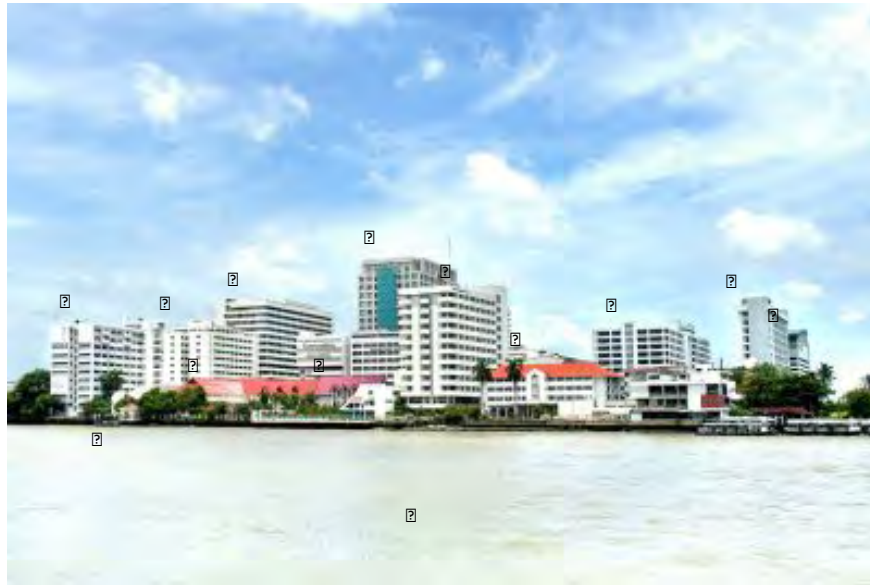
Figure 54: Development of Siriraj Hospital, 2005
