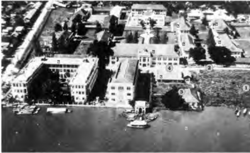
Figure 38: Development of Siriraj Hospital, 1948
