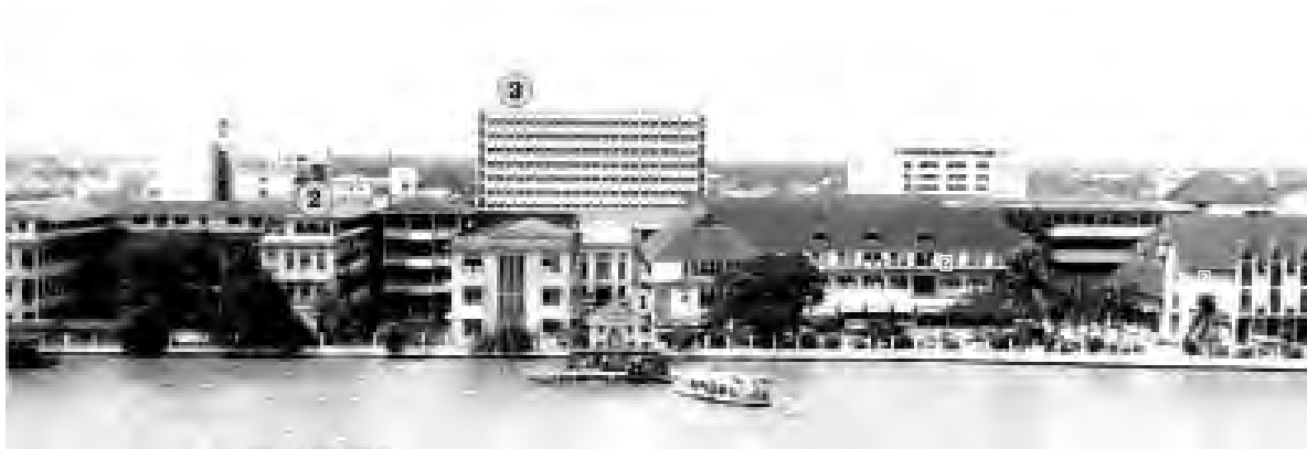
Figure 46: Development of Siriraj Hospital, 1971
