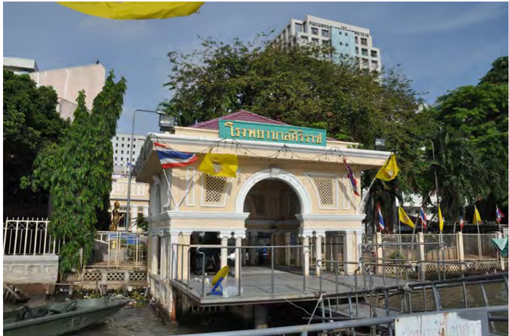
Figure 65: Siriraj Pier, built in 1923.
