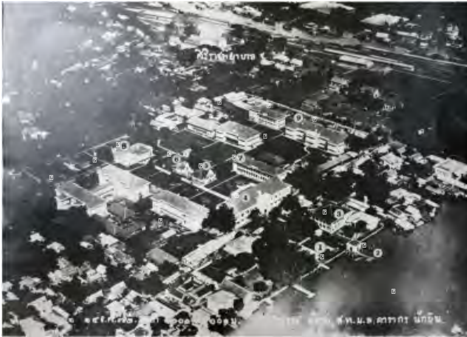
Figure 32: Development of Siriraj Hospital, 1929
