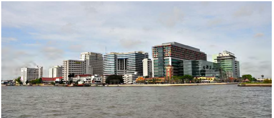
Figure 19: Siriraj Hospital 2012, form the junction of Chaopraya River and Bangkoknoi Canal
