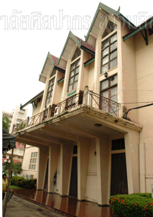
Figure 68: Rajapattayalai Auditorium (Source: Photo by Nantawat Sitdhiraksa, Febuary 29, 2012)
