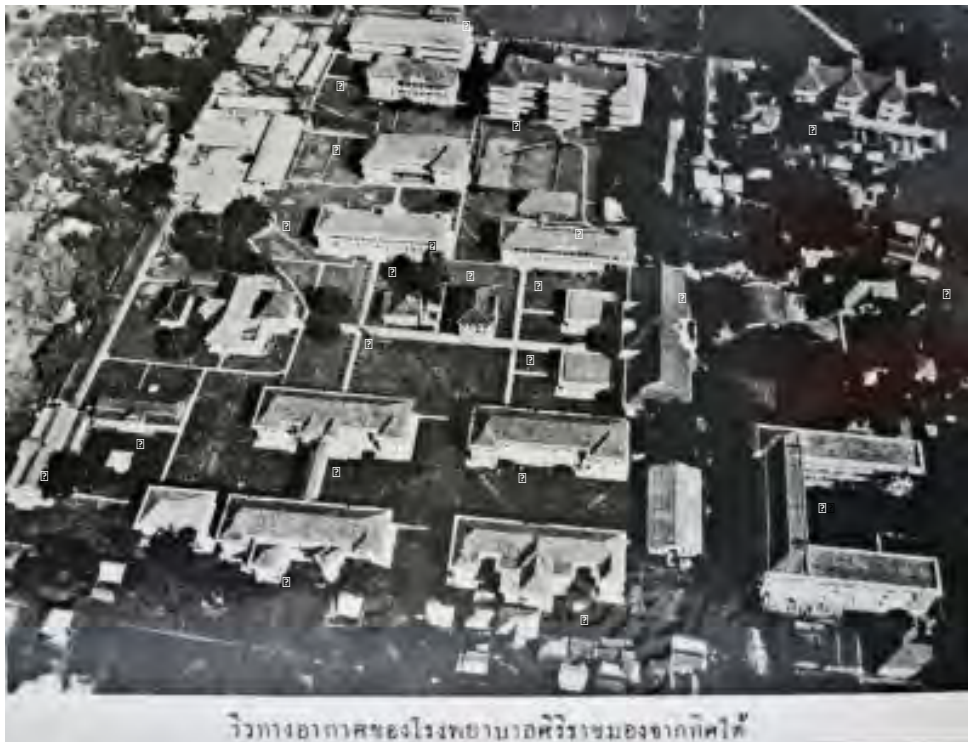
Figure 34: Development of Siriraj Hospital, 1935
