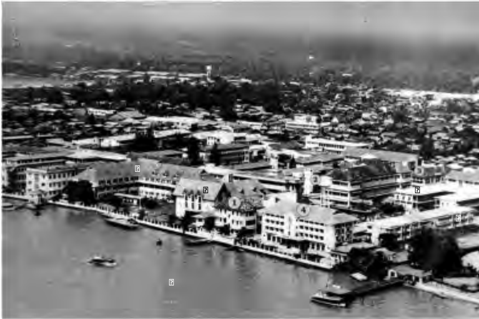
Figure 44: Development of Siriraj Hospital, 1964
