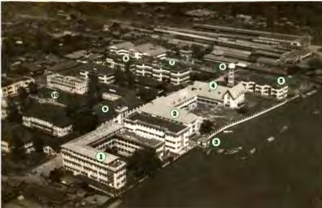
Figure 41: Development of Siriraj Hospital, 1957
