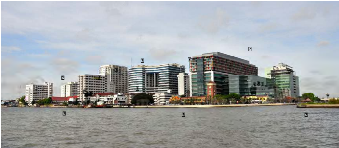
Figure 56: Development of Siriraj Hospital, 2012
