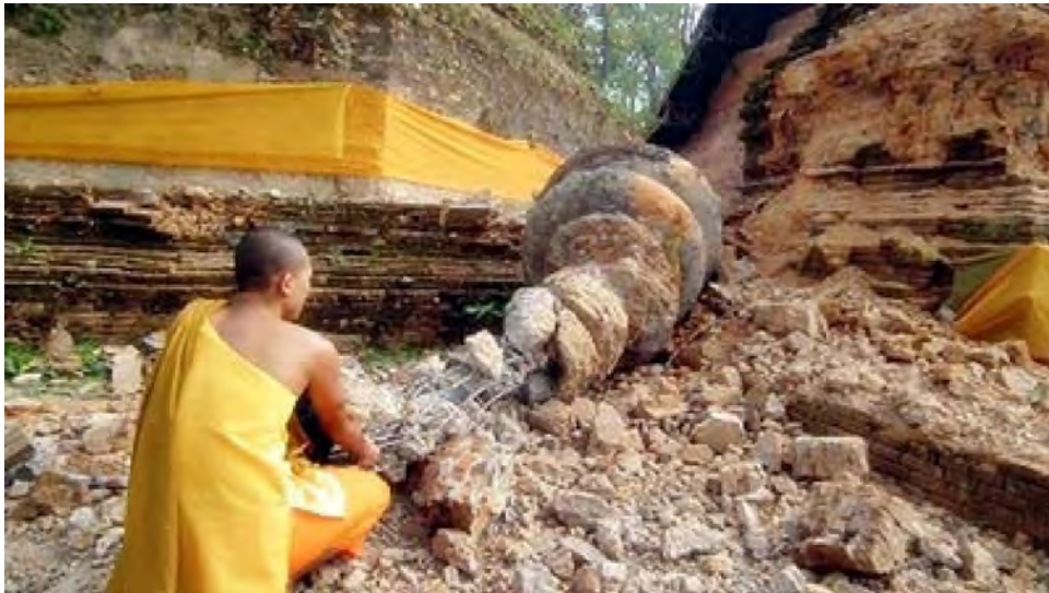
Fig. 39 Top of Chedi, heritage site in the northern of Thailand was collapsed from the earthquake on March 29th, 2011 reported by TTRWeekly newspaper
