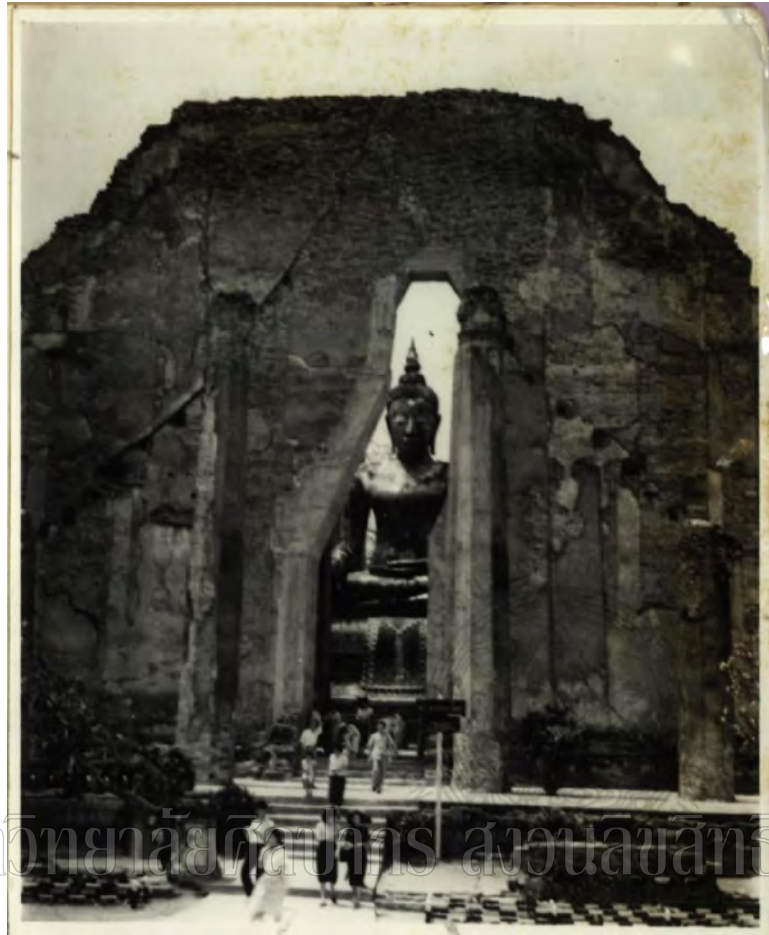
Fig. 64 Vihàra Phra Mongkhon Bophit in the past that without roof in deteriorate and ruined condition the entrance and platform in front of the Vihàra Phra Mongkhon Bophit (National Archives of Thailand).
