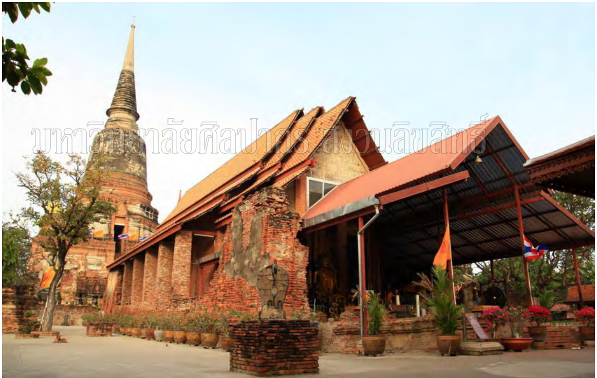
Fig. 42 The unfinished reconstruction Uposatha process on the original hall ordinary heritage monument east of Main Chedi, Wat Yai Chaimongkhon.
