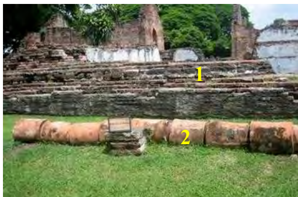
Figure 189 A water tank (1) and pottery water pipe (2) built in the King Narai Palace, Lopburi. The water pipe was constructed by a French engineer. They introduced waterworks between 1682-1684 starting at Lopburi and around 1685-1686 at the Ayutthaya palaces. Photograph by Phungwong, N. in February 2011.
