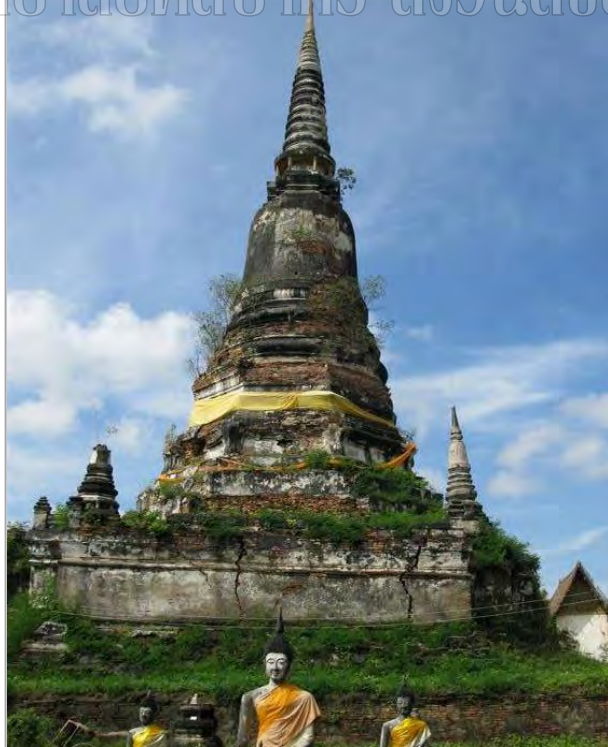
Figure 18 The Chedi of Wat Dusit, the area of the community which was existent before Ayutthaya period. This place was the home town of King Narai's wet nurse. Photograph by Phungwong, N. on April 29, 2009.
