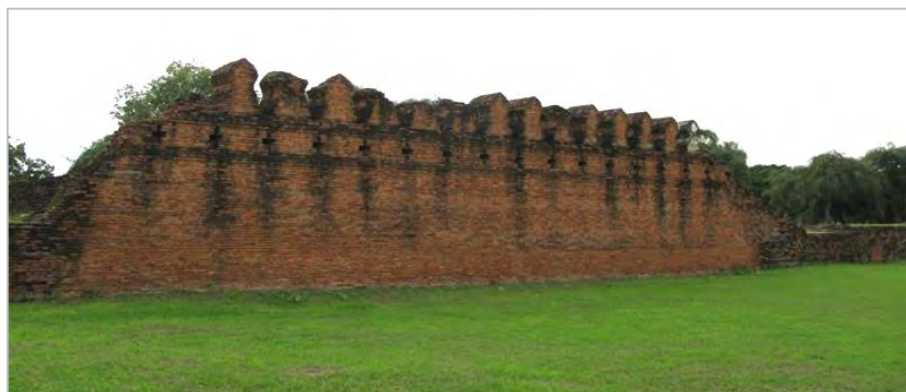
Figure 28 The remains of the Ayutthaya wall are seven meters high and ten meters in depth (foundation) in original formation. It is the last remain part of old city wall. Photograph by Phungwong, N. on May 1, 2009.
