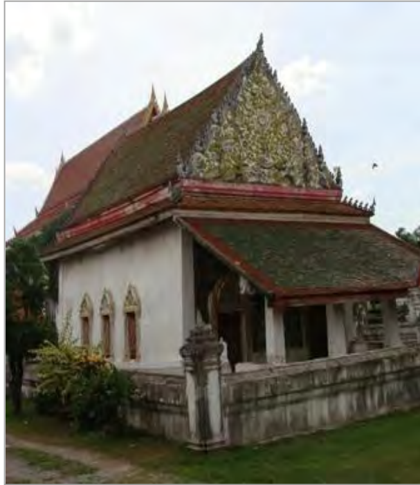
Figure 149 Wat Chotikaram in Nonthaburi was built in the Dutch or Vilanda style. The building is without columns and uses walls to carry the load. Mostly, local buildings in the central area received a very strong impact from the Dutch architectural style as it was simple and economical to build. The temple was built in the late Ayutthaya period. Photograph by Phungwong, N. on April 12, 2010.
