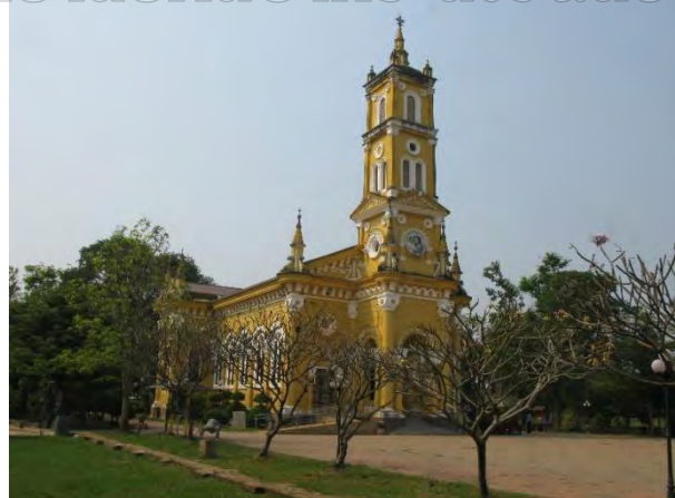
Figure 201 The new French church, Saint Joseph in present Ayutthaya province was built over the old foundation which some are remained in front of Church. The area has no excavation yet; today it is actively used by Thailand Catholic Mission. Photograph by Phungwong, N. on August 16, 2011.
