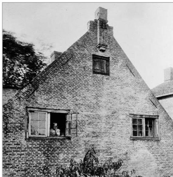
Figure 152 The Old Dutch house. Photograph shows the roof style “Dutch Gable” with roof slope less sharp than the Thai style where the roof slope is over 45 degrees. Photograph retrieved from http://www.andrewcusack.com on August 12, 2010.
