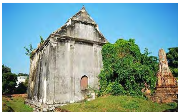
Figure 194 The small temple in Wat Prasri Mahathad, Lopburi, built with the influence of Gothic style but with fewer windows. It was call Ma-Ha-Aud style in Thai. This temple was built during King Narai's period. Photograph by Phungwong, N. in February 2011.
