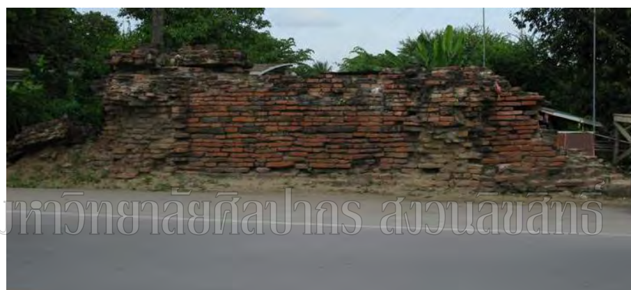
Figure 29 Above and below photograph shows the present day road around Ayutthaya Island built over the ancient Ayutthaya city wall. It was built in 1955 by a command of General Plak Piboonsongkram, Prime Minister of Thailand. Photograph by Phungwong, N. on May 1, 2009.
