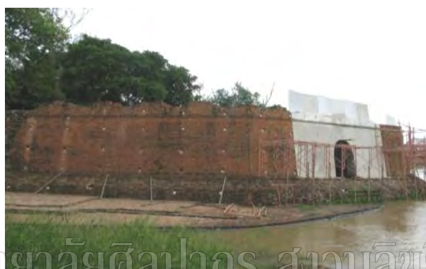
Figure 76 Pomphet (Diamond Fort). This fort was made from latalite and large bricks with a very strong foundation. This fort was the most important and largest among forts in Ayutthaya. In the beginning of the city, the city wall and fort was made from clay and wooden columns. It was reconstructed in bricks and stones during the reign of King Mahachakkaphat (1548-1568). He also built a large fort at the junction of the Parsak and Lopburi Rivers, Marhachai Fort to protect against enemies from the north. Photograph by Phungwong, N. on Jun 12, 2010.
