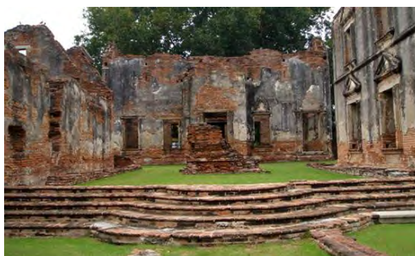
Figure 46 The front photograph of Vichayen's Home in Lopburi built in Renaissance-Thai style. It was built during the reign of King Narai. The European style mostly used bricks and mortar for the walls and foundation. For the roof used wood beam and terracotta tiles. This building represented a different between Thai and foreigners houses in Siam of Ayutthaya period. This photograph by Phungwong, N. October 23, 2010
