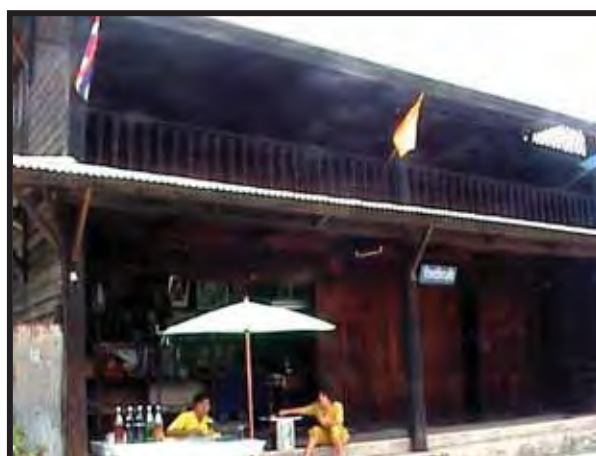
a. Sriyapai House (Southern Architecture)
