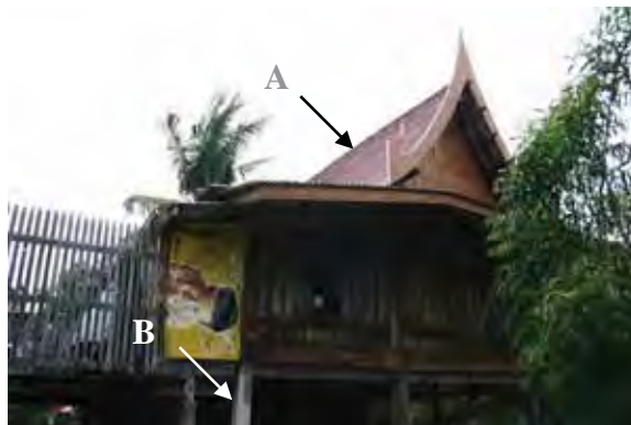
Figure 44 The traditional Thai house found in Pakkran village with changes at roof cladding (A) and ground level columns (B)
