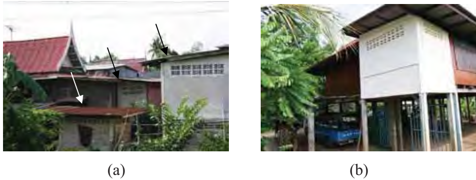
Figure 69 External and internal bathrooms
