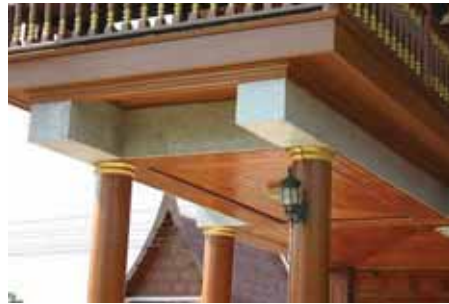
Figure 75 Concrete structures at ground level
