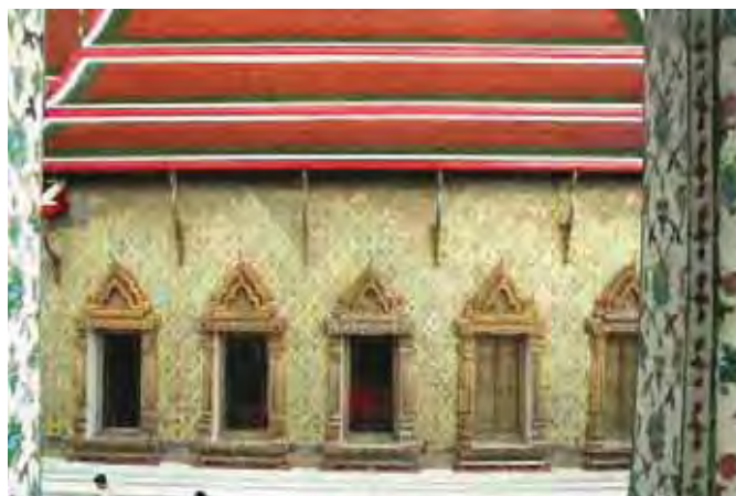
Figure 34: Window and outer wall Photograph by: Kanjanaphorn Polprateep : June, 2008
