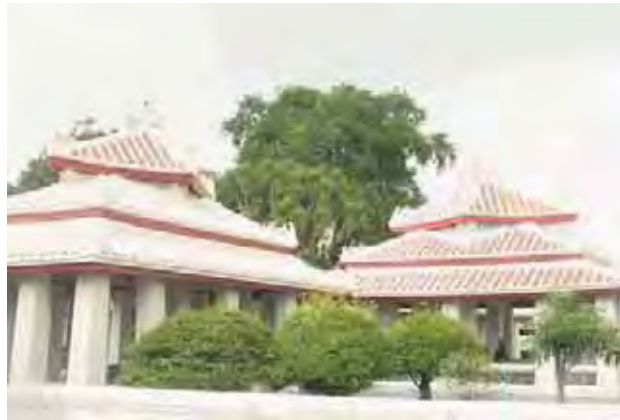
Figure75 : Riverside pavilions Photograph by: Kanjanaphorn Polprateep : June, 2008
