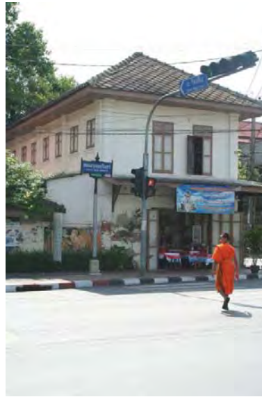
Figure 106: The existent old building
