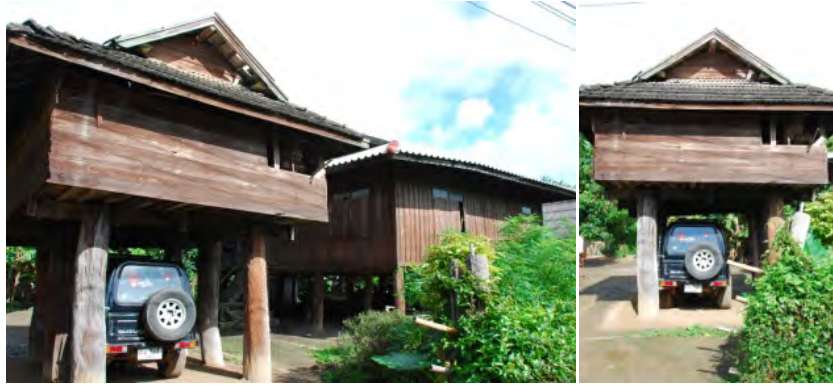
Figure 24: Former rice storehouse made from teak wood which is belonged to one of Mae Chaem's family. (Viamlin V., August, 2008)
