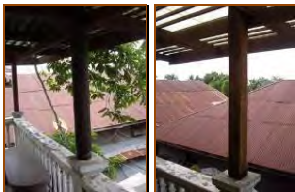
Figure 31-32: Poles at 3 rd floor (left) The original pillar; (right) a new pillar
