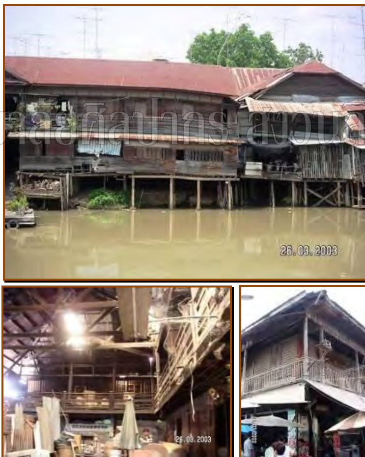
Figure 13-15: Most of the shop-houses in Soi 1 and 2 were in poor condition, pictured in 2003 (before renovation)
