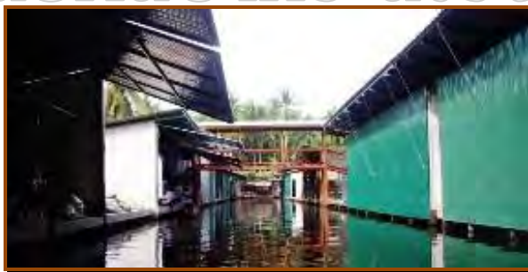
Figure 233: Many vacant shop houses (new project) along 'Ton Kem' canal
