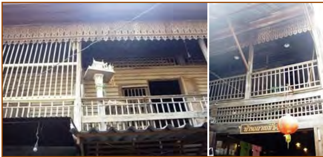
Figure 17-18: Carved wooden curtains (khanompang khing) from the era of Kings Rama V and VI
