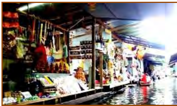
Figure 232: Row of one storey shop houses along 'Ton Kem' canal
