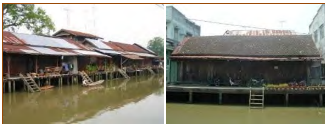
Figure 86-87: houses were in poor condition, imaged in 2000
