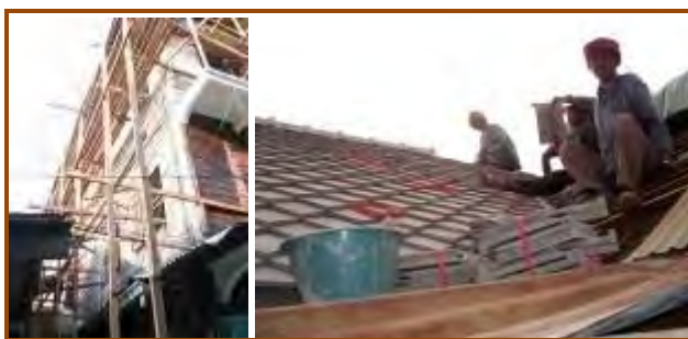
Figure 66-67: the repair of Baan Khun Jamnong
