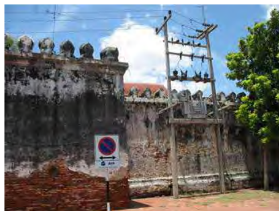
Fig.54 Constructions block the view of the significant places (Pic. From survey)
