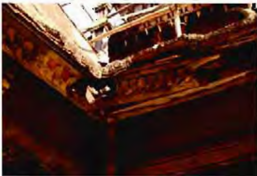
Figure 10: Eave and roof valley
