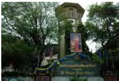
Figure 131: Bell tower of the Saint Francis Xavier church
