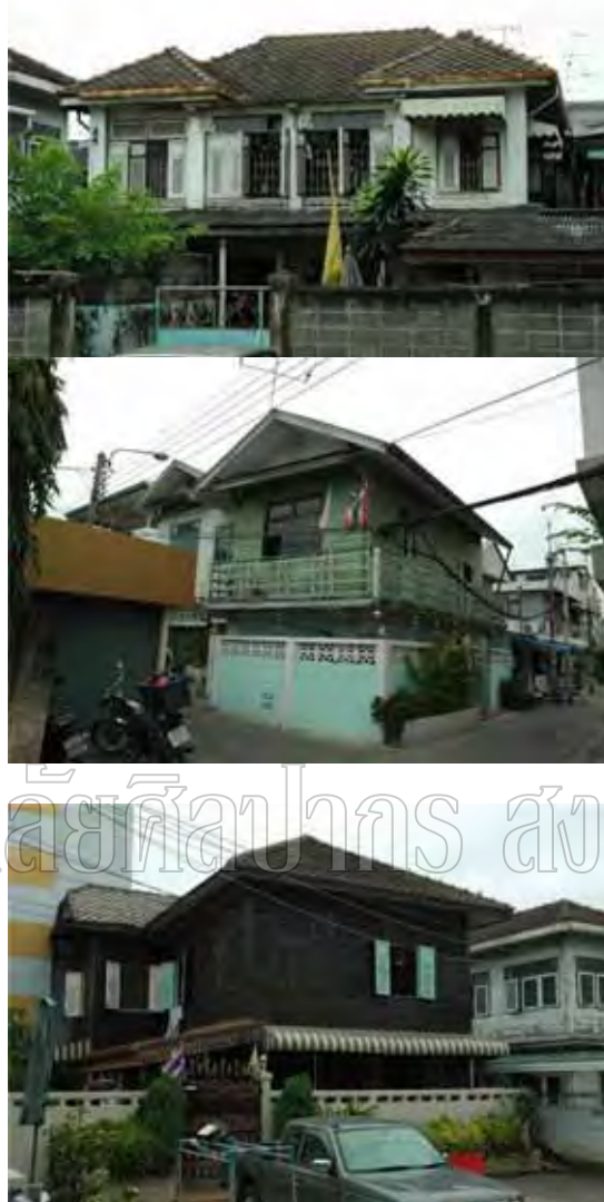
Figure 141-143: Traditional houses at the community (Source: Author)
