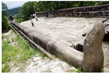
Figure 31: Naga bridges are causeways lined by stone balustrades shaped as nagas. (Source: Thai FAD 2008)
