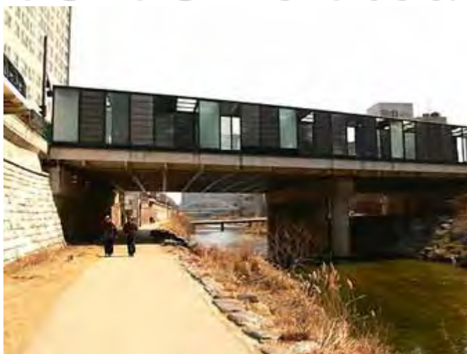
Figure 82: Hwanghak-gyo (Photo taken by Noh, Jang Suh on March 7, 2009)
