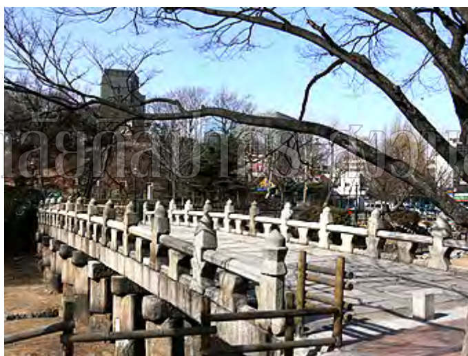
Figure 50: Original Supyo-gyo at the relocated site (Photo by Noh, Jang Suh)
