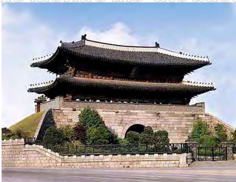
Figure 154: Namdae-mun (south gate)
