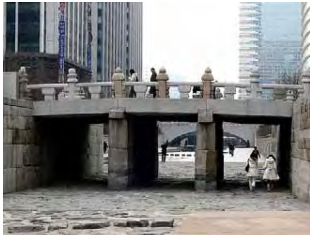
Figure 28: Restored Gwangtong-gyo (Photo by Noh, Jang Suh. The bridge is relocated 155 meters away upstream from its original location.)
