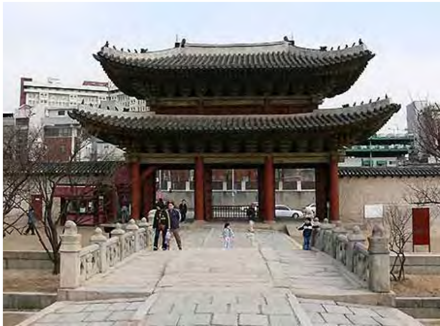
Figure 141: Main gate, Changgyeong-gung (Photo by: Noh, Jang Suh)
