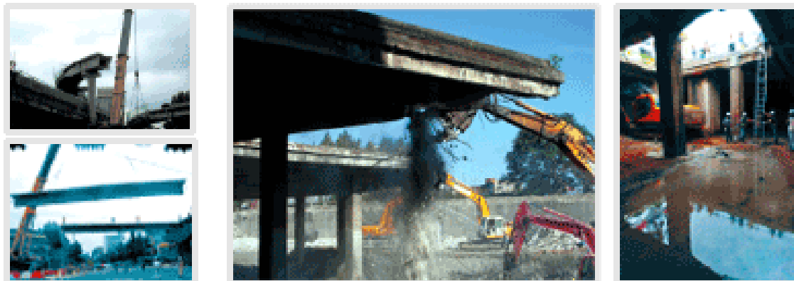
Figure 18: Photos of removal work
