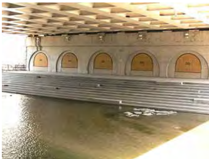
Figure 90: Floodgate (Photo taken by Noh, Jang Suh on March 7, 2009)
