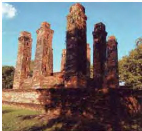
Fig. 91 Close-up of the square columns at Hor Thewalai Mahakaset Phimarn
