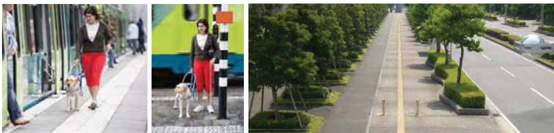
Figure 320: Tactile paving surfaces can be used to convey important information to visually impaired pedestrians about their environment.
