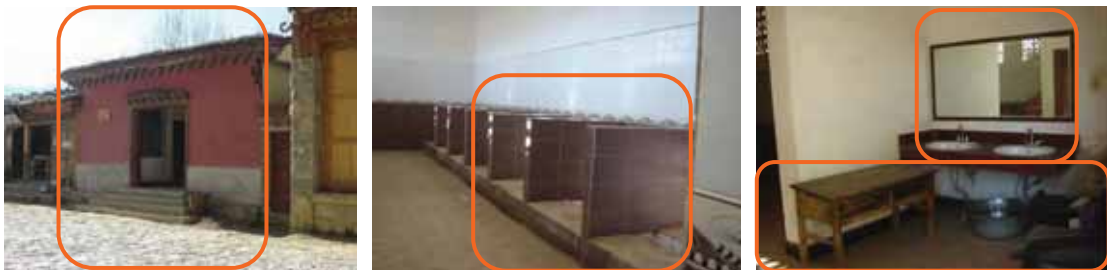
Figure 178: No. 4 Along two facing walls, there were concrete platforms about eight inches high. These were divided into "stalls" with low walls.
