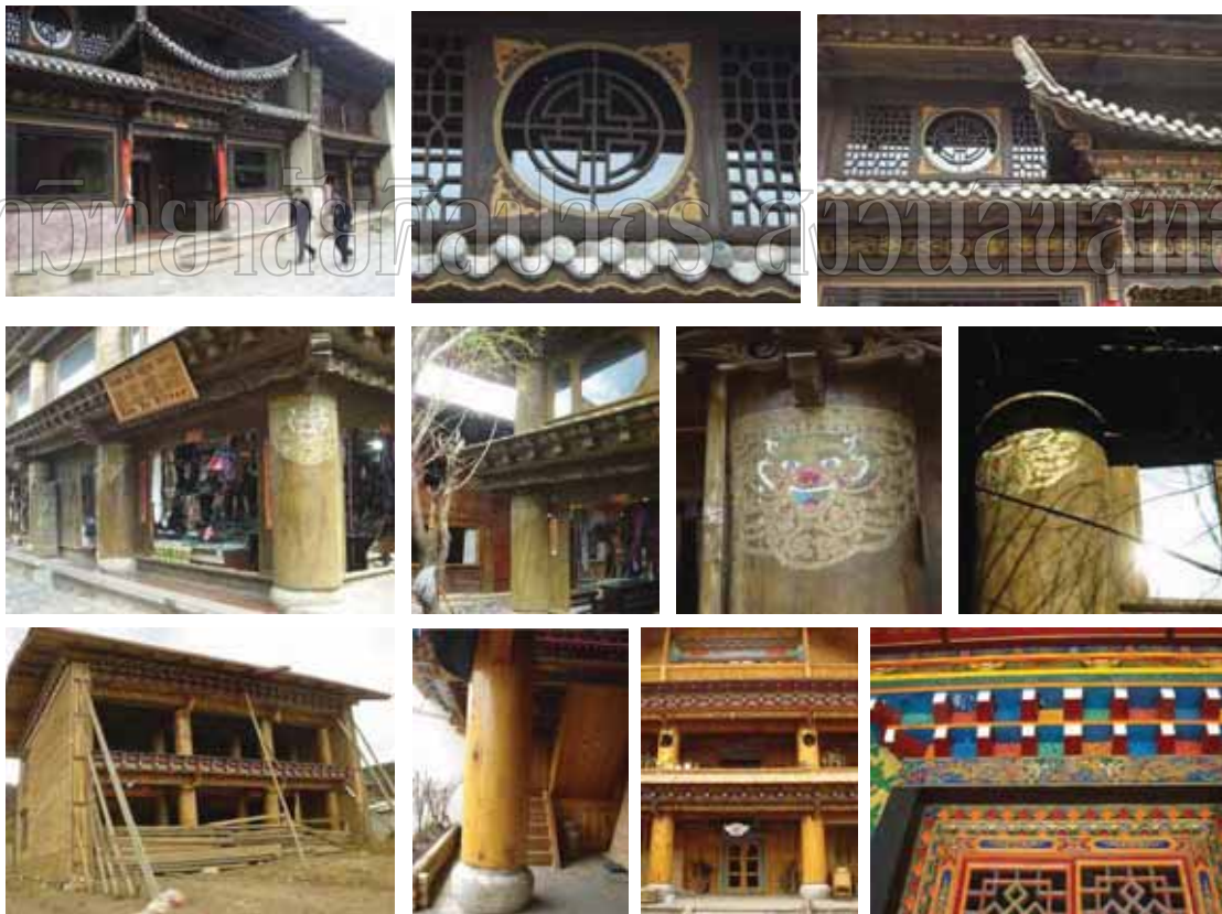
Figure 138: The most unusual feature of Tibetan architecture is many of the houses and monasteries are built on wood imported and used abundantly for housing. Horizontal timber beams support the roof, which in turn are supported by wooden columns.
