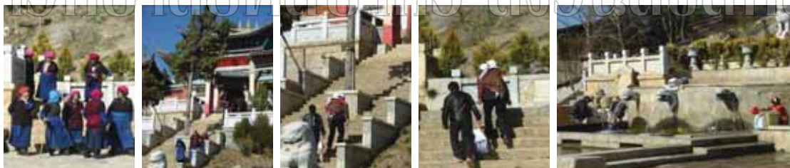
Figure 165: Stage 1: Ground floor the first level, the stairways are located in front of the main entrance from height staircase up to higher stages. A grand staircase leads up to the second stage. The open-air steps are deep and do not have handrail on left/ right sides going up. It has landing space in single floor level. A portable ramp would not be able to apply for wheelchair ramp. It is difficult to climb and can be dangerous because of the risk of tipping backwards. Visual perception on a panoramic image with the “normal” distance perception standard.
