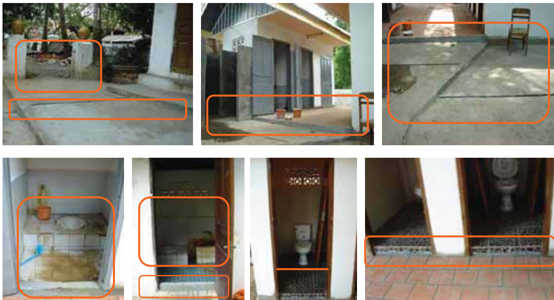
Figure 127: Small aisles keep the pathways free where people walk, a few raised floor steps toward making people access to public toilets. Step free access is also required between ground floor and flooring around the toilets. The biggest obstacle a wheelchair user is entry door and turning space in the toilet room.
