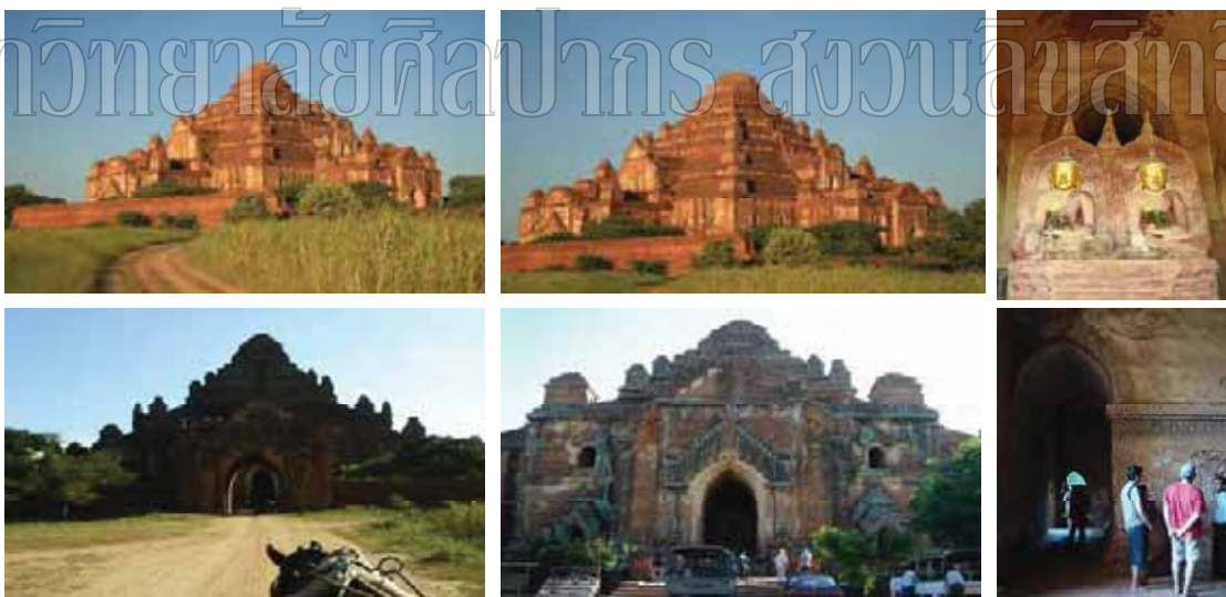
Figure 233: Dhammayangyi Temple is one, among the four significant monuments of Bagan. Dhammayangyi Temple is the most massive structure in Bagan, which has a similar architectural plan to Ananda Temple.
