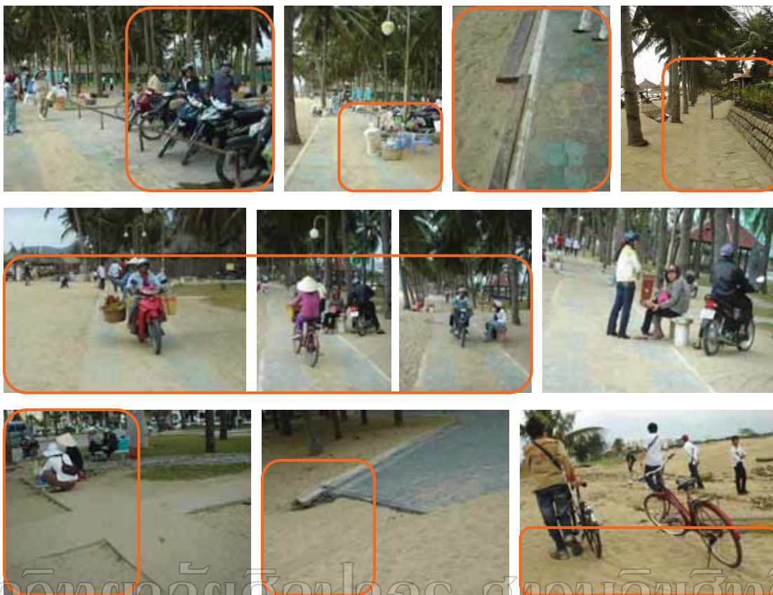
Figure 300:- The material for sidewalks is built on firm hard surface and not slipping, but too high curbs, changes in level, and no slopes or ramp.
