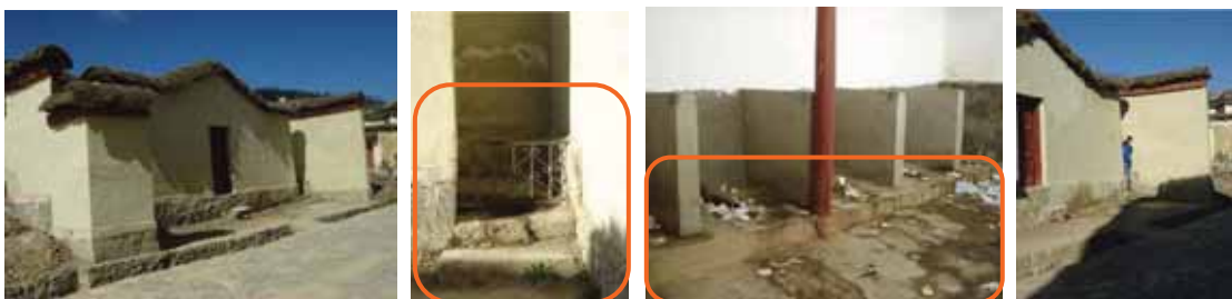
Figure 179: No. 5: Public toilet facilities. These are basically concrete rooms with no roof. In each stall cut into the rectangle platform. Under this hole, is a concrete slab tilted downwards towards a trough. The idea is that whatever people drop through the hole will roll or slide down the slab into the trough, which will then be flushed with water once in awhile.
