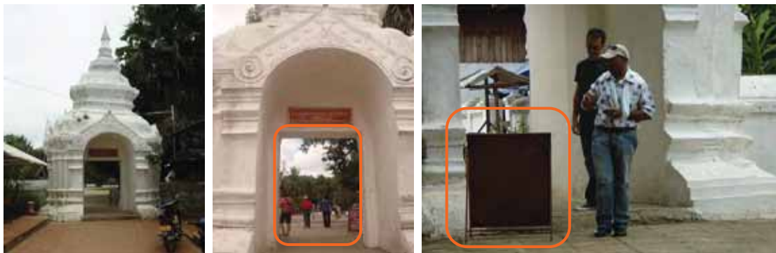
Figure 116: Bold identification of gatehouse wide transfer space to the temple visitor and wheelchair accessible. The freestanding signage is blocked the main gate entry to the temple. It is obstacle to blindness and vision impaired people.
