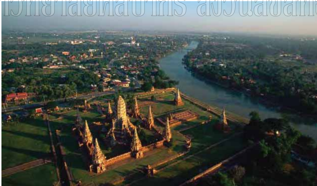
Figure 208: Chai Wattanaram Temple lies on the western bank of the Chao Phraya River.
