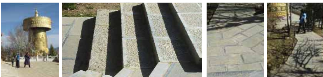
Figure 167: Stage 3: There are small steps and short distance access into the largest golden prayer wheel in the world. Floor material made from unpolished-granite terrace around the golden prayer wheel, Material friendly made it easy to walk around, but does it only clockwise, as religious tradition dictates.
