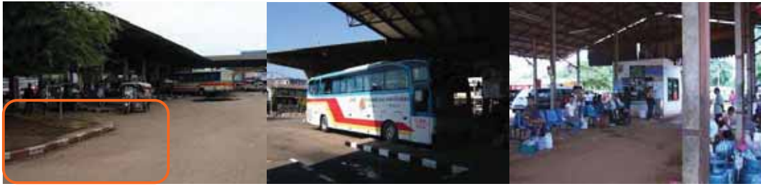
Figure 86: Coach Station in Nong Khai province Thailand sale tickets from Thailand to Vientiane. Public transportation needs to be accessibility for person with disabilities. The low-floor bus and street level are adjacent to a platform the different height as the bus floor. The waiting area is very convenient and more spatial for all passengers walking throughout area.
