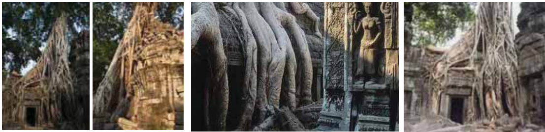
Figure 265: The Ta Phom Temple roots growing over temple, which disrupt and waste statues and walls, and huge trees beat the heads of stupas.
