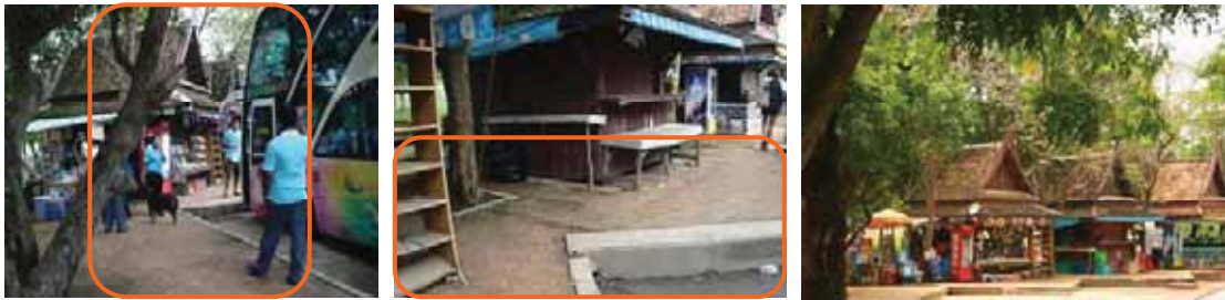
Figure 211: This sidewalk width allows enough space for two pedestrians' comfortably walking side-by-side, but flowerbeds, furniture, umbrellas and vendors make it difficult for a wheelchair and pedestrians pass through. Narrow sidewalk is a result of obstructions.
