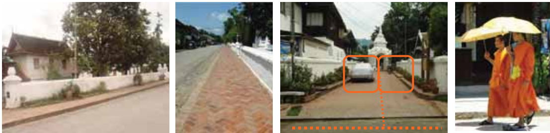
Figure 111: Entrance B Access from Sakhalin Road: Designation parking spaces are not provided for disabled drivers and passengers. Sidewalks are public for the use of all citizens. The vehicles are parking on the sidewalks. People with vision impairment can not see the obstacles.
