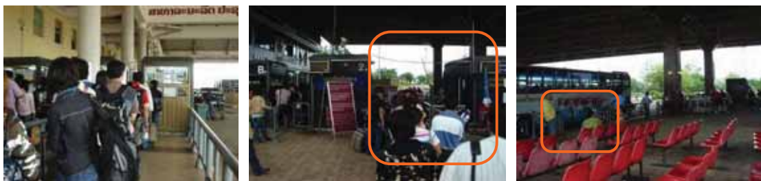
Figure 88: Thailand-Lao immigration checkpoint in Nong Khai to Vientiane. The parallel narrow entry/exit rail bars are obstacles for pass through. The gateways of the immigration service are not for people with disabilities. The ground floor level has different height between step and floor bus.
