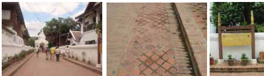
Figure 115: Welcoming gateway to the destination access to the temple. The Xieng Thong Temple blended curbs in tooled terra cotta between Main Street and sidewalks and pavement of the UNESCO historic materials.
