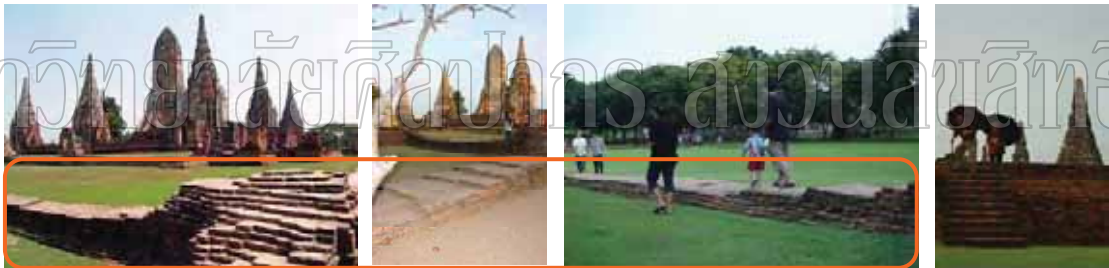
Figure 221: Visitors had difficulty walk through some steps, slopes average walk on sidewalk and courtyard. Now people walk over the heritage places and destroyed heritage fabric.
