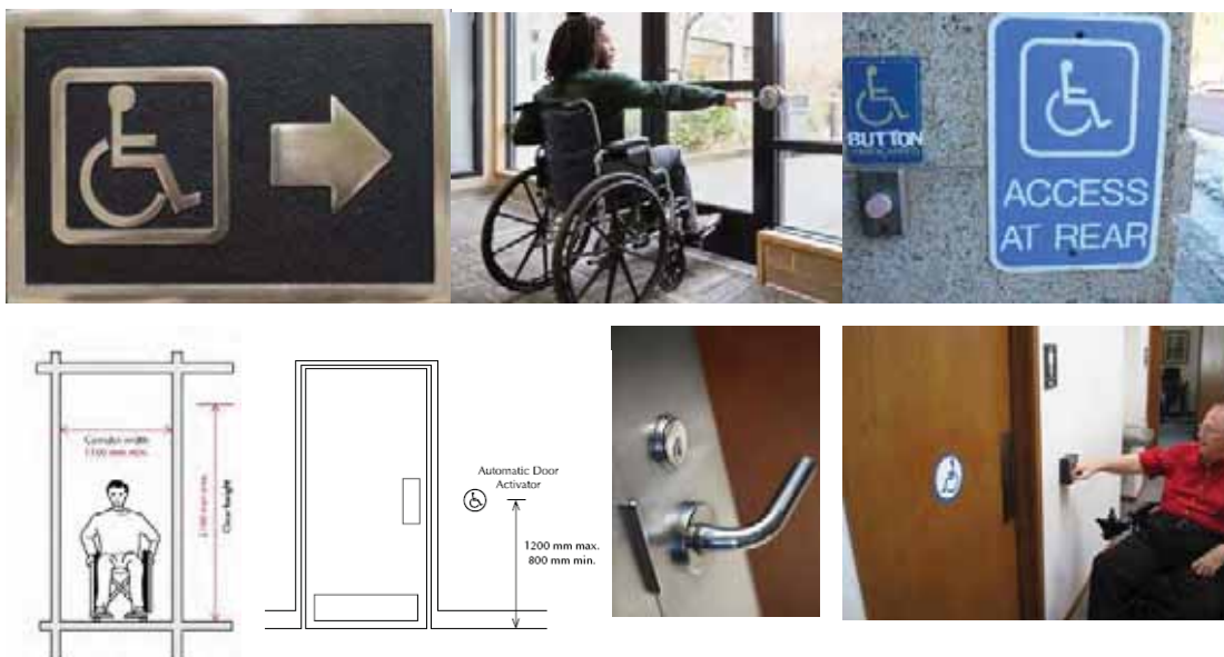
Figure 316: Automatic door openers are recommended wherever possible.
