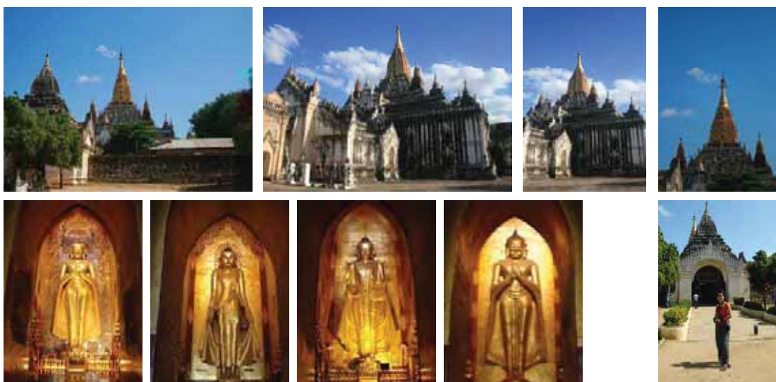
Figure 231: Ananda Temple is considered to be one of the most surviving masterpieces of the Mon architecture. Also known as the finest, largest, best preserved and most revered of the Bagan temples. During the 1975 earthquake, Ananda suffered considerable damage but has been totally restored.
