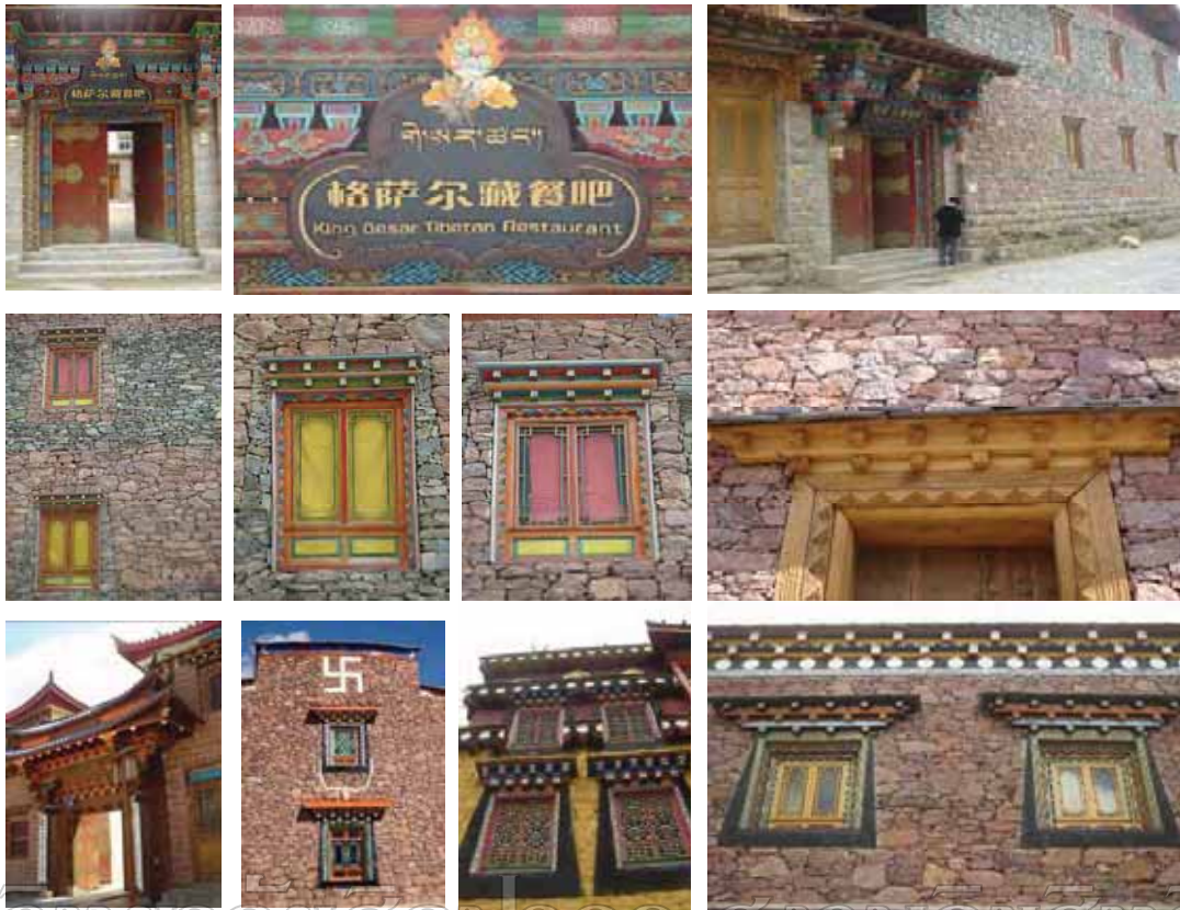
Figure 140: Houses constructed with earth, stone and wood in their surrounding villages, looking like a castle, are colloquially called “castle” by the local people.
