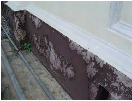
Fig.98 Splash of rain as source of decay Photo by: Supachokeauechai, T.
