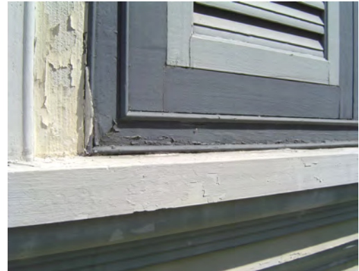
Fig.104 Crazing of paint from weathering and humidity penetration Photo by: Supachokeaueychai, T.
