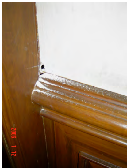
Fig.109 Wooden walls are drilled for insecticide injection Photo by: Supachokeaueychai, T.
