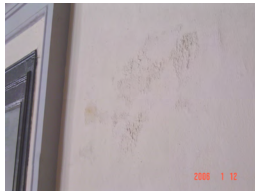
Fig.95 The evidence of paint blistering Photo by: Supachokeaueychai, T.
