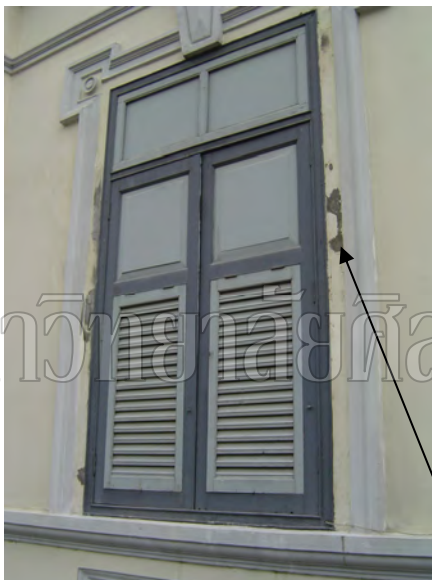
Fig.103 The decay of sill and jamb from rain water Photo by: Supachokeaueychai, T.
