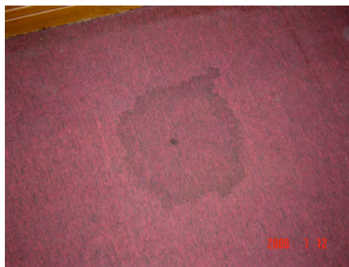
Fig.102 Carpet flooring as source of fungi and black spots Photo by: Supachokeaueychai, T.
