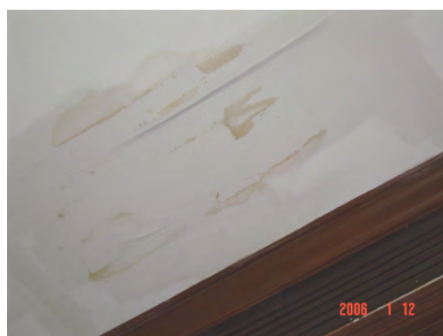
Fig.108 Fungi spot at the interior gypsum ceiling Photo by: Supachokeaueychai, T.
