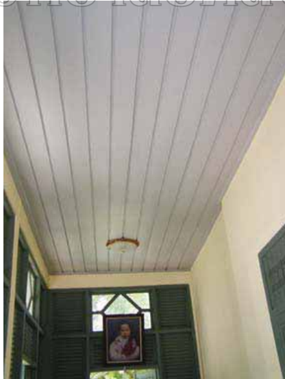
Figure 114: The ceiling in regular style. It made from timber planks
