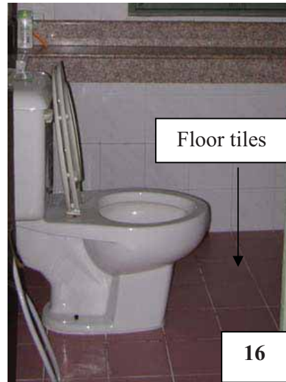
Figure 111: The new ceramic floor tiles of the toilets
