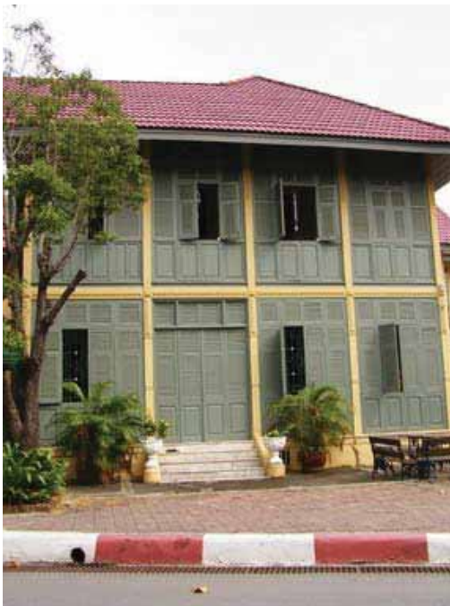
Figure 100: The west is connected by an inside road.
