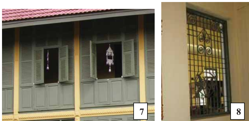
Figure 105: General condition 5, two styles of windows
