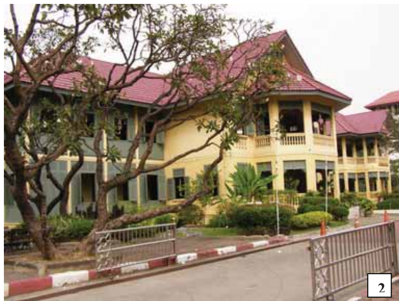
Figure 102: General condition 2 The architectural style of Saisuddha – Nobhadol Building is colonial style.
