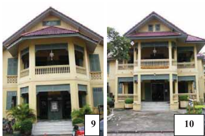
Figure 106: General condition 6. Two porches with marble stairs functioning as the main entrances in the south. Above each porch, there is a terrace covered with different styles of roof design.
