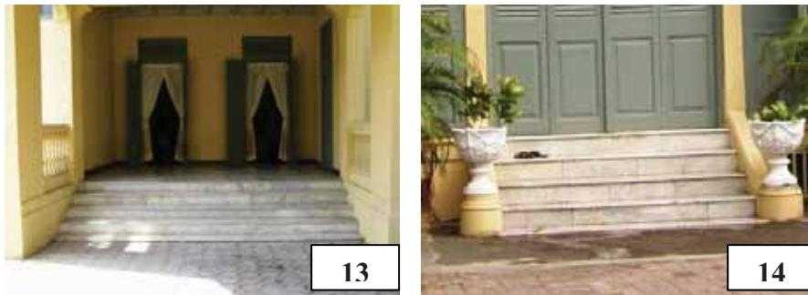
Figure 108: A marble stair in the east
