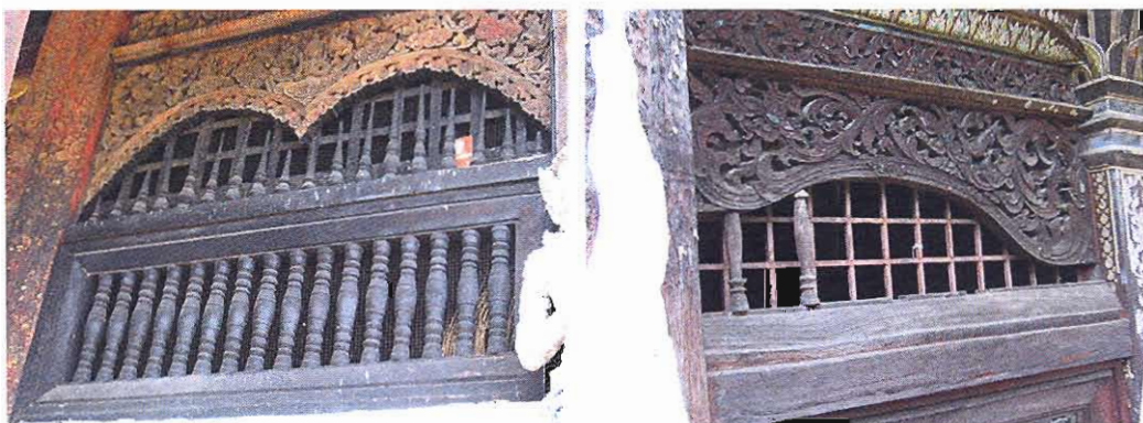
Figure 34 showing carved wood ventilation grilles of Wat Buak Kok Luang (left) and Wat Ton Kwen (right) Source: author, 26 August 2006
