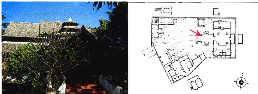
Figure 14 showing architectural detail of the main building Source: author, 15 November 2006
