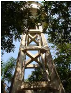
Figure 75 Water supply system (taken by Muangyai, N, 24/01/09)
