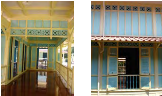
Figure 99-100 The use of modular system throughout the building (taken by Muangyai, N, 29/01/09)
