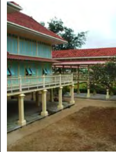
Figure 175 The palace's systematic design (taken by Muangyai, N, 06/04/08) - From the exterior, the appearance is that of a two-storey building. Each section has an opening for ventilation covered with framework in Art Deco Style.
