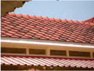
Figure 96 Rhombus-shaped roof tiles (taken by Muangyai, N, 29/01/09)
