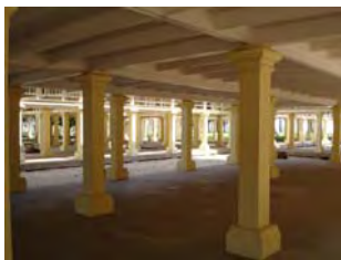
Figure 103 Concrete stilts arranged in modular system (taken by Muangyai, N, 29/01/09)
