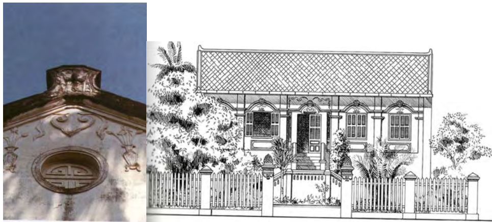
Figure 83 Lao colonial house, 1930. Ban Phone Heung. Renovated in 1990. Private house.
