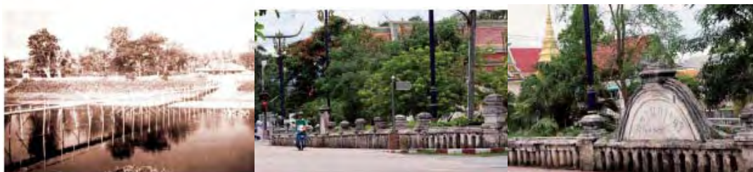
Figure 54 Krung Sri Bridge, from past to present
