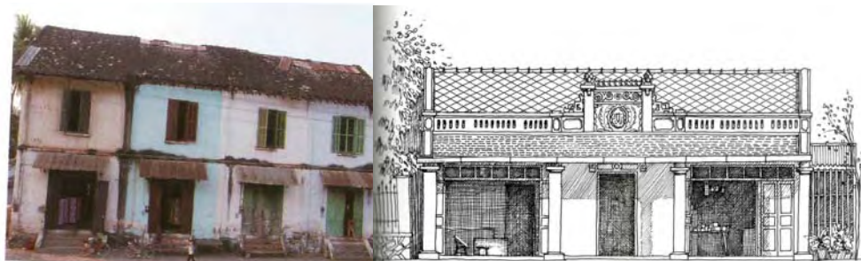
Figure 84 Shophouse, 1923. Ban Pa Kham.
