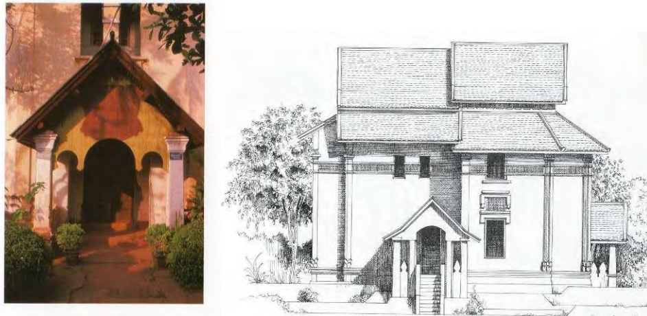
Figure 80 School principal's residence, 1922
