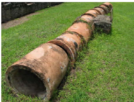
Figure 9 Terra cotta pipelines
