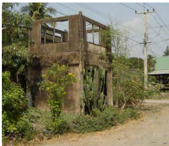
Figure 32 Two-storey railway substation
