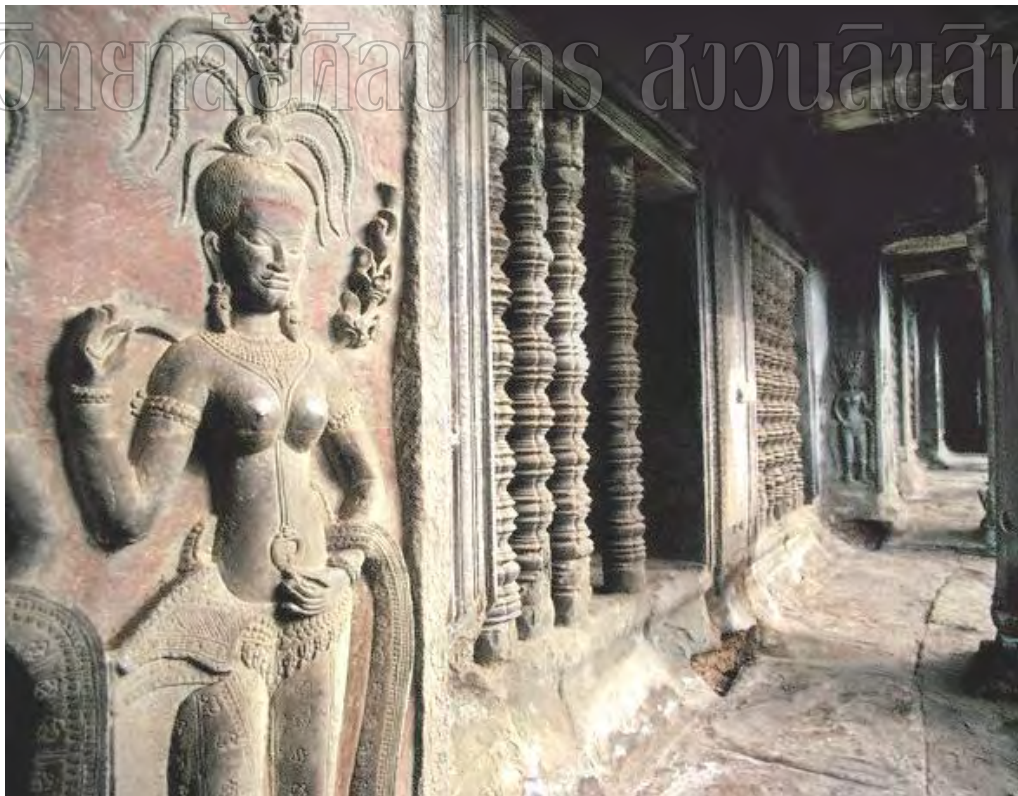
Figure 24 Details of Khmer architecture; “false window” balusters, stack construction, surface decoration, www.corbis.com
