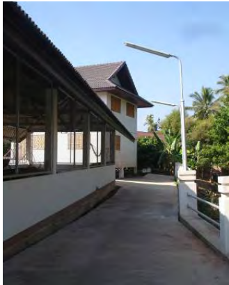
Figure 118 : Collapsed buildings after the opening of the OTOP fair : the racing boat building
