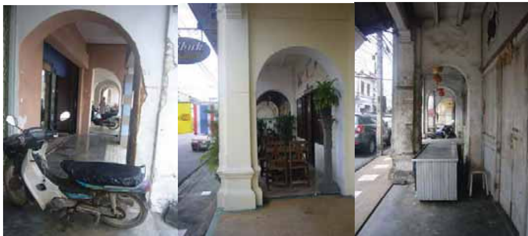
Fig. 55 The continuous front arcade known as a 'five-footway'. Photographs taken by author on 14 December 2007
