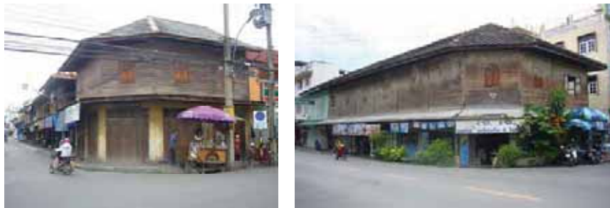
Fig. 73 Shophouse characteristics in King Rama V's reign. Photographs taken by author on 5 May 2007
