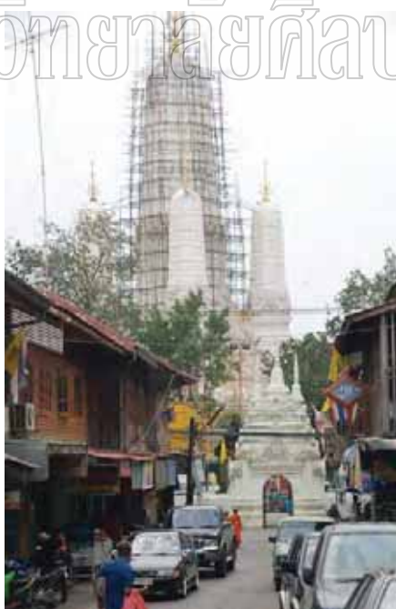
Fig. 76 Wat Mahathat, a landmark of the community and Phetchaburi city. Photograph taken by author on 19 August 2007.
