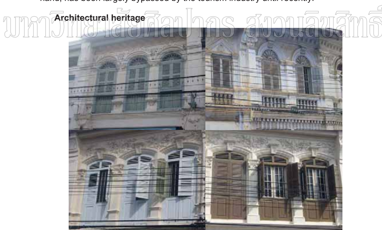
Fig. 52 Cultural built heritage of Phuket that still remain the full richness of their authenticity. Photographs taken by author on 14 December 2007
