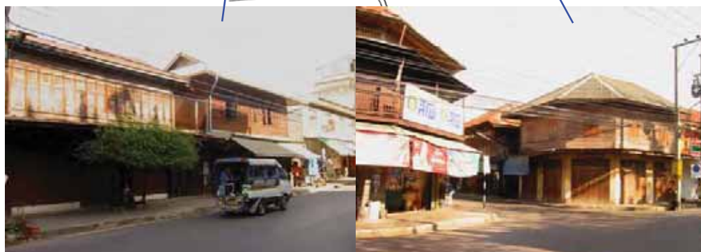
(Damnernkasem Rd. shophouse type C)
