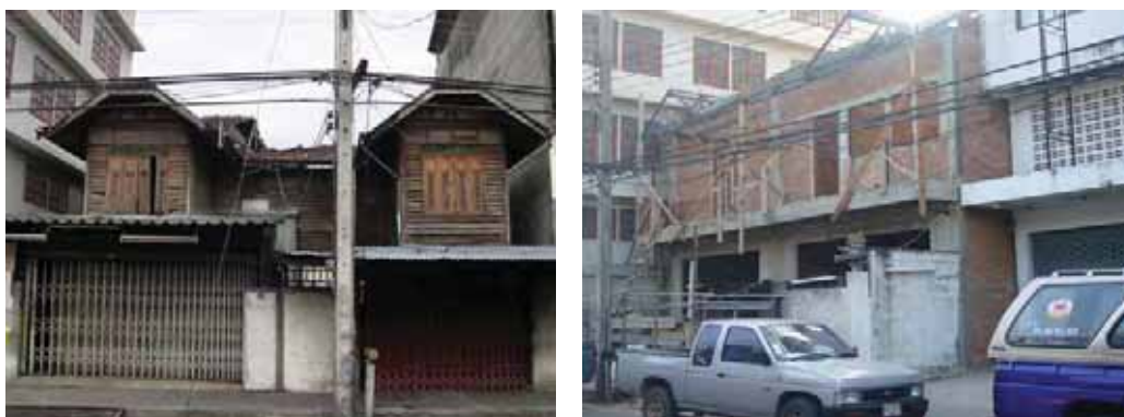
Fig. 2 The poor condition shophouses are demolished and made way for monotonous “modern” buildings. Photograph from survey on May, 2007 then December, 2007 taken by author
