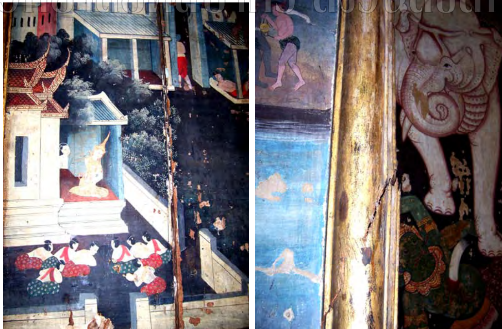
81. There some damage on the wooden materials. The doors and window have split and are scratched. The gold parts are rubbed. Photographs by Bussayamas Nandawan
