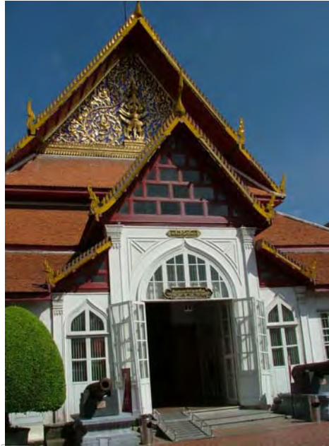
42. The front view of Phra Thinang Sivamok Pimann. The main entrance is a large wooden door that folds up vertically with glass panes. The door's strength is weak.
