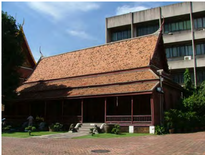
46. The Tamnak Dang building or Red House at National Museum, Bangkok, Thailand
