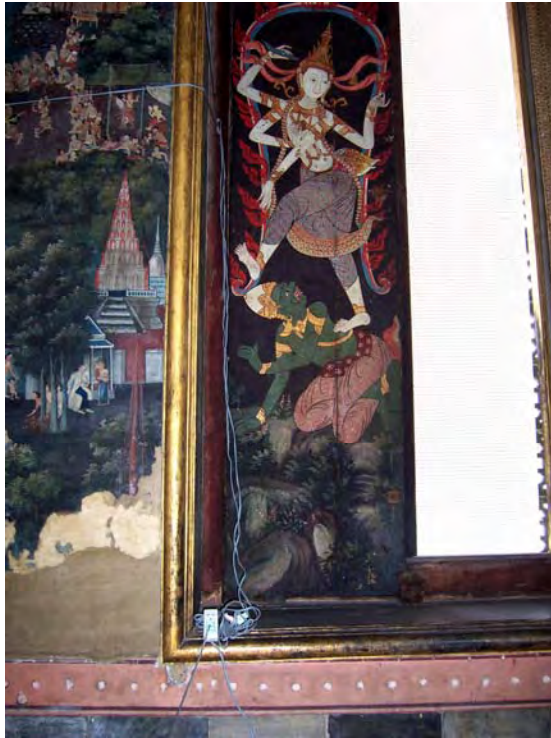
82. The electronic wires are in a mess. They jump from one window to another window. Vulgar nails were put on the wooden window panels for hanging the wires.
