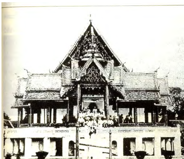
23. The building called Phra Thinang Kochakam in the front of Phutthaisawan Chapel
