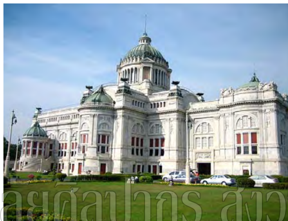
Figure 151: The Ananta Samakhom Throne Hall signifies the full westernisation of Siam under King Chulalongkorn.
