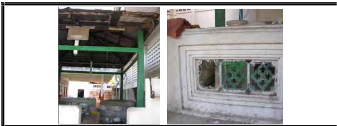
Plate 48 The existing condition of the well's pavilion
