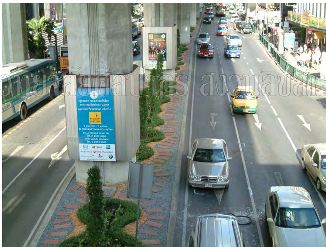
Figure 19: Looking eastwards on Rama I: most vehicles run westward except the bus while concrete columns for the BTS sky train occupy the middle of road, by the author, on 12 th August 2006.
