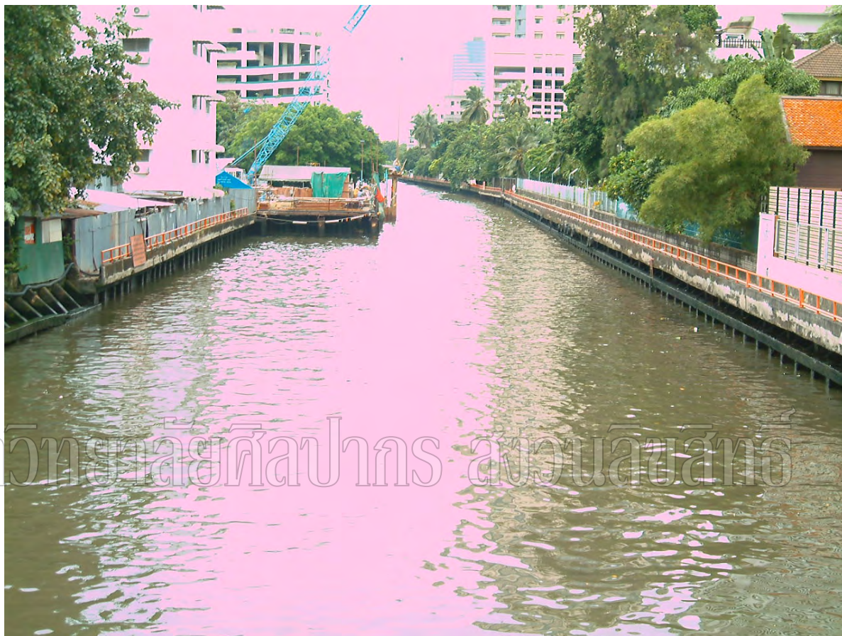
Figure 30: Passage of Khlong San Saeb, looking eastward from the bridge at Sukhumvit soi 3 (Nana), by the author, on 12 th August 2007.
