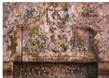
Figure 83: Pediment of the Bhavalai depicting Shiva Nataraja on an elephant back, which is rarely found (Source: TAT, 2004b)
