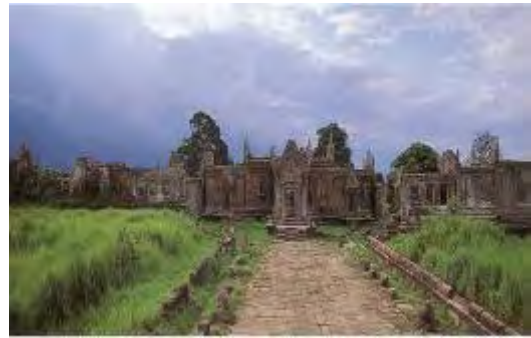
Figure 79: The Mahamandira which was built into a large rectangular hall (Source: TAT, 2004b)
