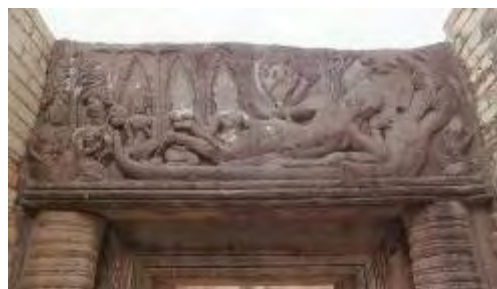
Figure 76: Lintel of the principal tower depicting reclining Vishnu, Vishnu Anantasayin (Source: TAT, 2004b)
