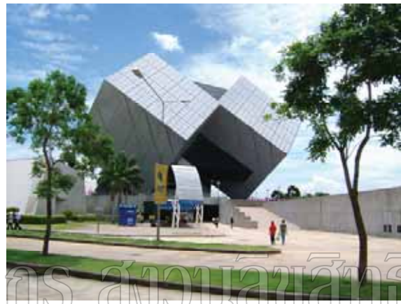
Figure 49 The construction of NSM.
