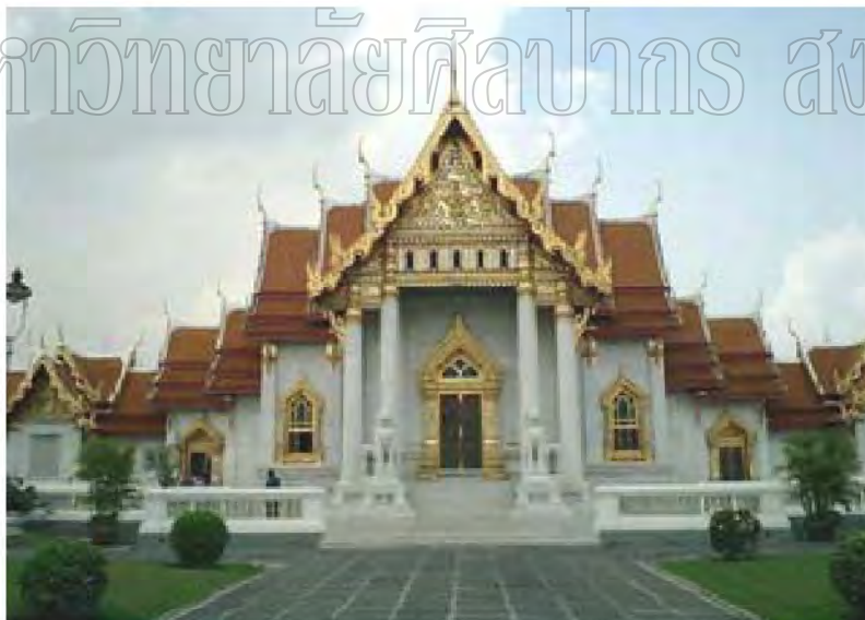
Figure 24. The main chapel at Wat Benjamabopit or the Marble Temple, Bangkok, creating a Western architectural concept on the traditional functions of Siamese monastery.
