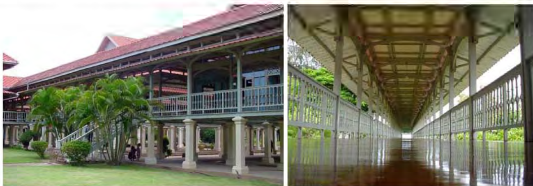
Figure 4. (Left). The design of the Beachfront Palace based on a modular system in response to the opening for tropical climate. Figure 4. (Right) A long walkway of the Beachfront Palace possessing horizontal elements. Space exposing to the sea breeze for whiling away the time and relaxation. (Photograph: Korrachai Lekpetch).
