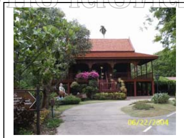
Figure206: Library near the entrance of the park
