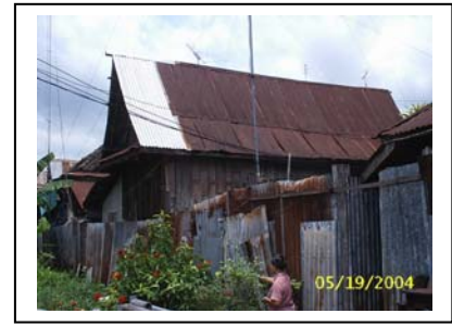
Figure94: Corrugated iron roof on traditional Thai style house
