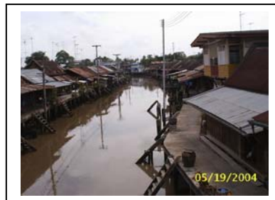
Figure 99: Landscape of Amphawa canal is lined with single, 2- storeys and twin wooden house
