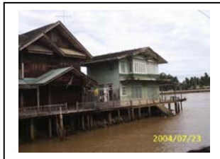
Figure 42: Contemporary Thai house at Amphawa canal mouth
