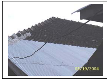
Figure126: The mixture of terracotta tile and corrugated iron sheet roof
