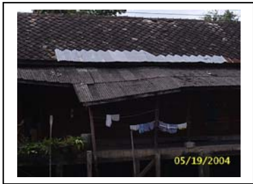
Figure101: Original terracotta roof with additional corrugated iron sheet in repairing
