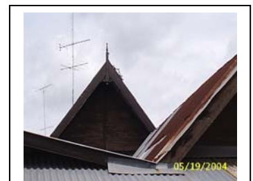
Figure 92: Decoration on the pointed part of windbreak
