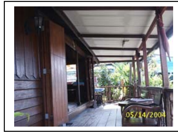
Figure146: Entrance (view from the other side)
