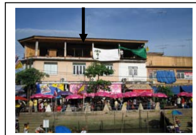
Figure 278: Inappropriate height of new intervening building
