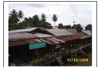
Figure 100: Roofscape of terrace of single house with coconut tree behind
