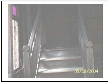
Figure72: Wooden staircase inside the 2-storeys house
