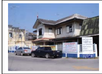
Figure63:This building was Chinese language school in the past, but present it is an office of Amphawa Municipality.(Contemporary Thai house)
