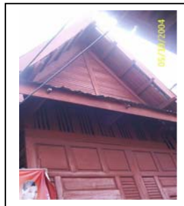
Figure76: A low pitched roof above projecting eaves
