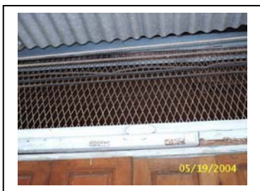
Figure101: Original terracotta roof with additional corrugated iron sheet in repairing
