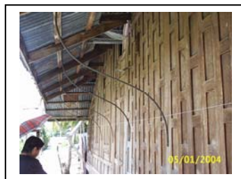
Figure132-134: Wooden and metal bracket found at the riverside shop-house at Amphawa canal
