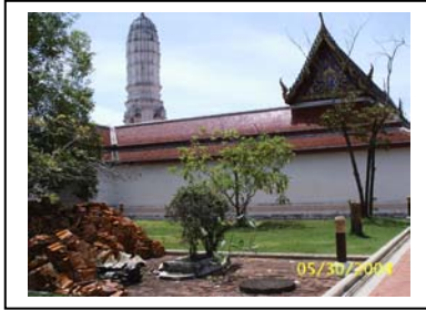
Figure191: Right: view of Vihara from Prachasret Road
