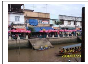
Figure 43: concrete building at the Amphawa market
