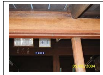
Figure156: adjoining point on the ceiling
