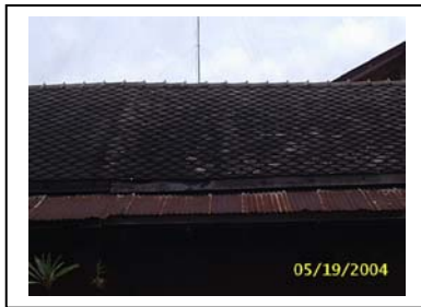
Figure95: Terracotta tile roof cover a terrace of single house
