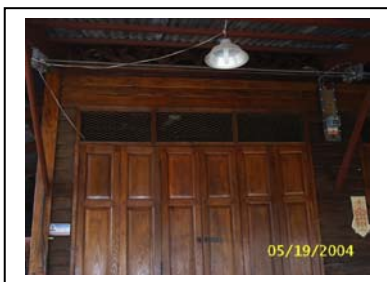
Figure104-111: Various styles of ventilation panel at top of various designs of folding door
