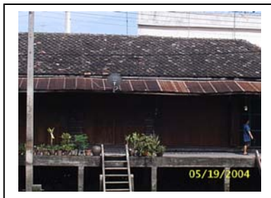
Figure137: A small ladder for water transportation use
