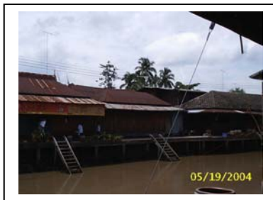
Figure98: A single house covered by corrugated iron sheet and terracotta tile roof
