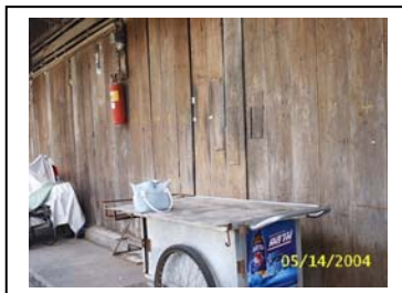
Figure140: Wooden panels of door still are found in Amphawa community, somebody said this is a former creation before becoming folding door. (They put hinge into each of wooden panel.)
