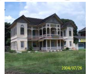
The ancient building located in the boundary of this temple
