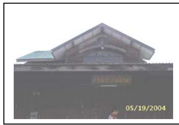
Figure85: Front view of roof
