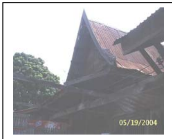
Figure75: A high pitched roof and its decorative gable finials in stead of Ngao style
