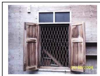
Figure79: Wooden window with metal sheet inside
