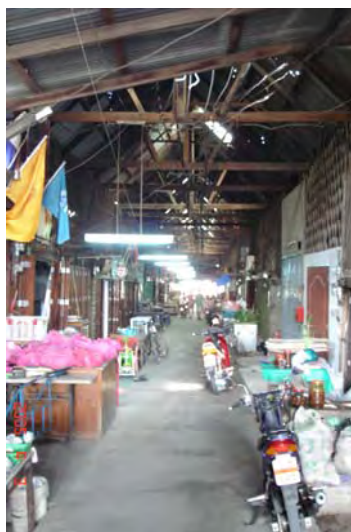
Figure 4: The high roof and wooden structure is commonly used in Don Wai River Market for ventilating heat and providing air flow throughout the day, especially in the hot and sunny day during summertime
