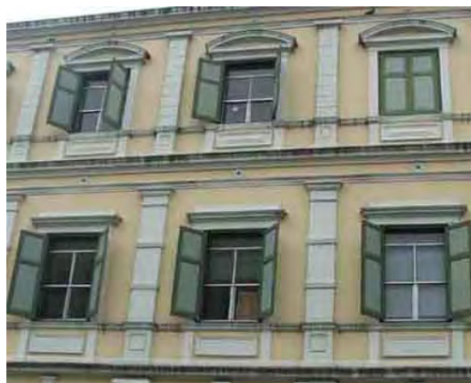
Figure 18. Aluminum window frames are installed / Building A.
