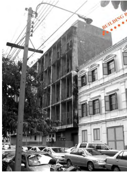
Figure 9 and 10. Building C / Ministry of Defence. (photo: Mr. Korn Prabhasabhakdi, 2005)
