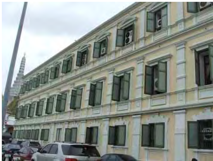
Figure 14. Main building / Ministry of Defence.
