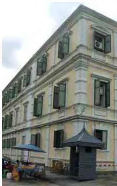
Figure 17. New booth was built in front of the building / Building A.
