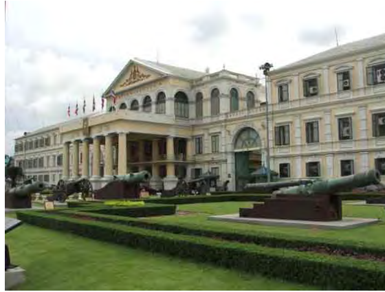
Figure 6. Building A / Ministry of Defence. (photo: Mr. Korn Prabhasabhakdi, 2005)
