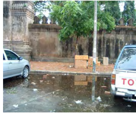
Pollution in the parking near the northern wall Figure 1
