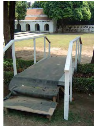
Synthetic material covered passage way Figure 3
